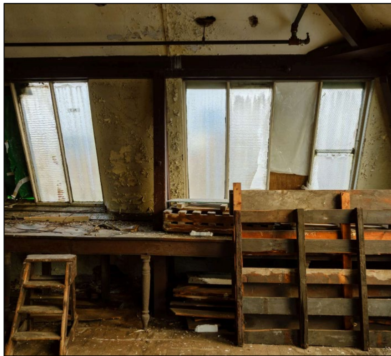
Figure 2.4: Existing Interior of the Site (4 th Floor Level)
