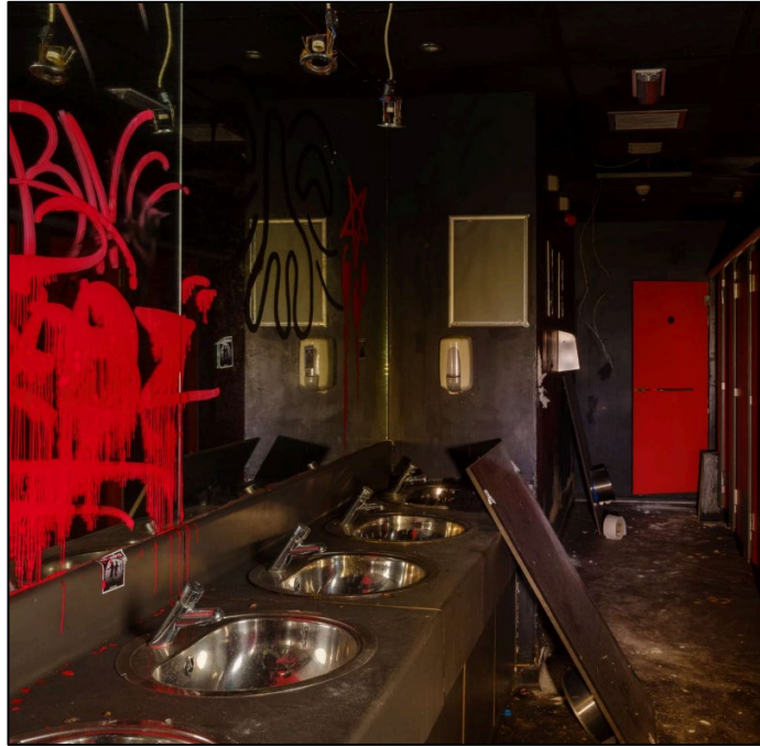
Figure 2.3: Existing Interior of the Site (Basement Level)
