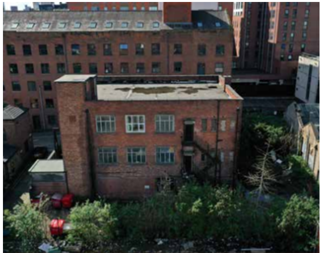
Figure 2 – Rear elevation with Beehive Mill behind
