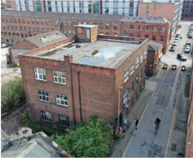
Figure 1 – Front and northwest side elevation
