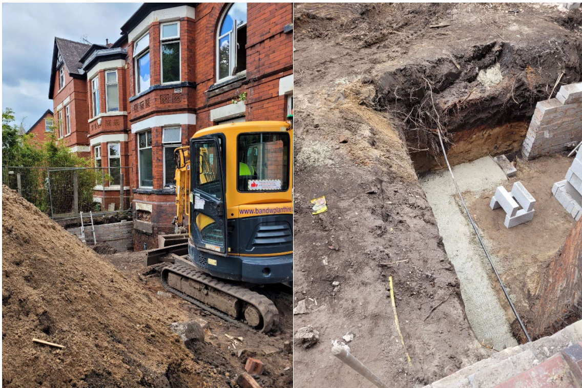
Front elevation digs to prepare for new lightwells to the principal elevation. Existing clean sand base.
