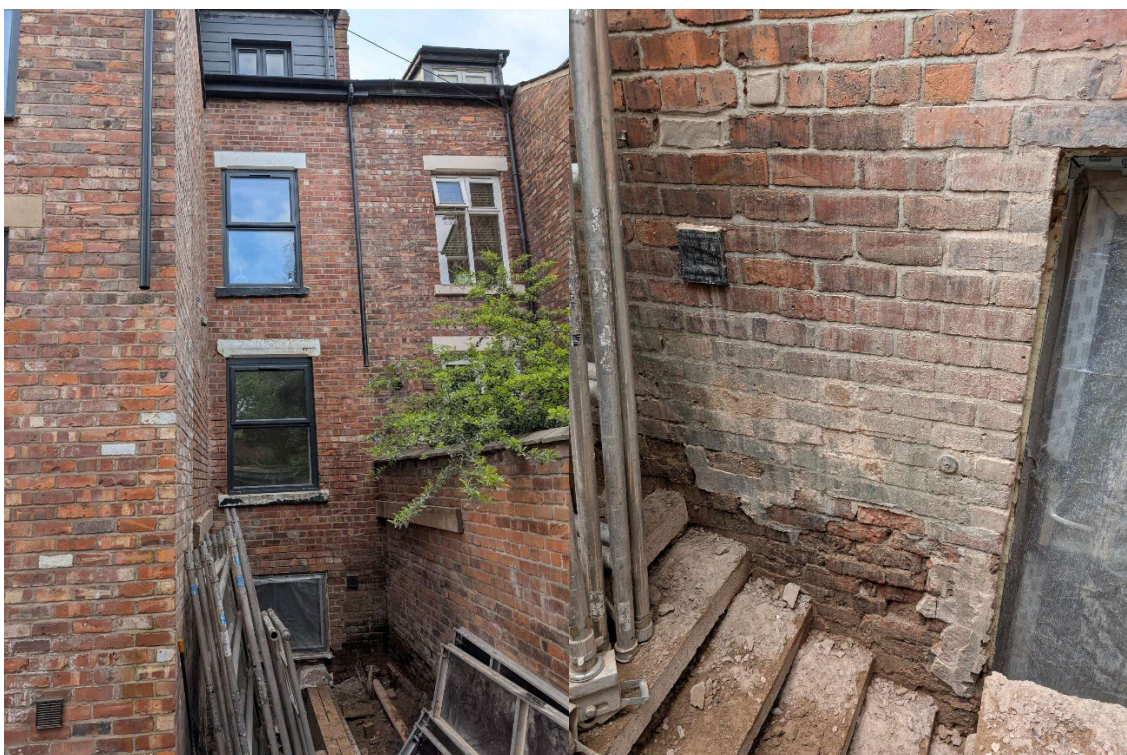
Rear elevation: Very little groundworks and ground movement was required to the rear elevation. Existing use was of car parking area and rear access retained.
