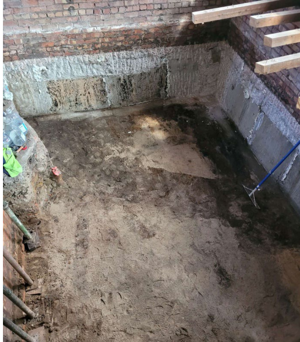
Internal dig to prepare for new slab. Existing clean sand base.
