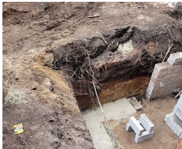
Ground removal to the front elevation to form lightwells. (Additional photos in Appendix B)
