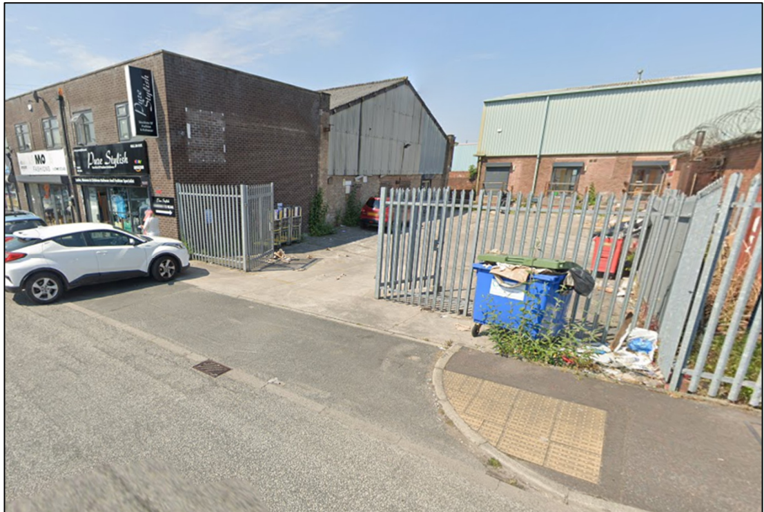
Figure 2.3: Existing Access off Bradstone Road
