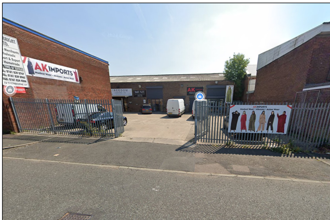
Figure 2.4: Existing Access off Sherborne Street
