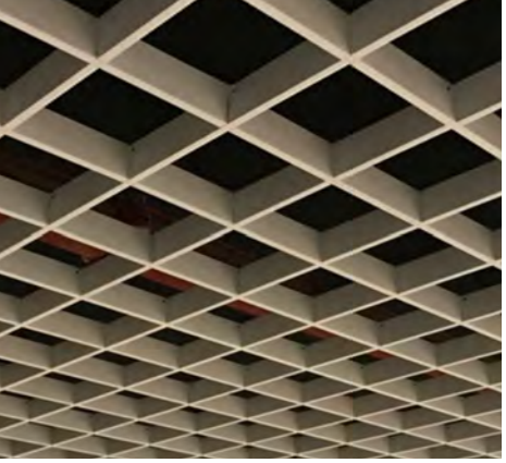
CEILING FINISH - SPEC: KNAUF, CELIO, RAL 1013
