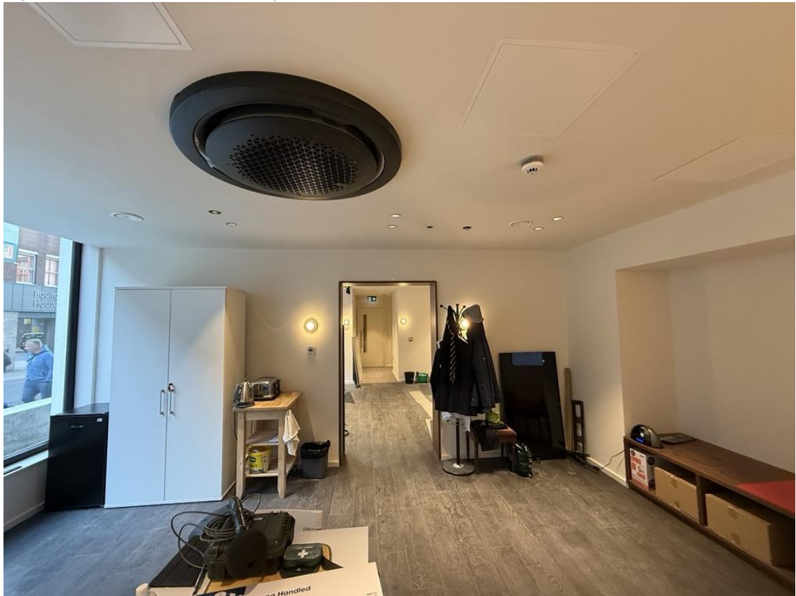
Figure 2.1: Plasterboard Ceiling to Gym
