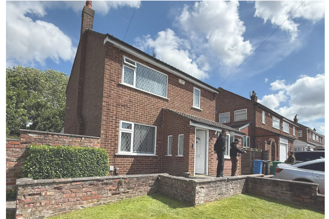
34 Dunnisher Road. Photograph from the front of the property.
