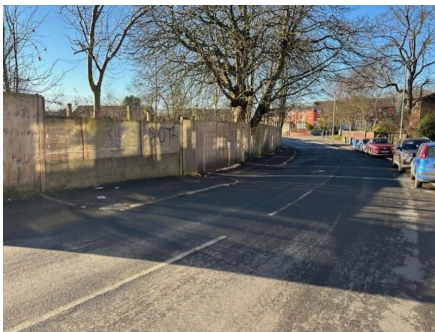
View of site looking north-west along Church Lane
