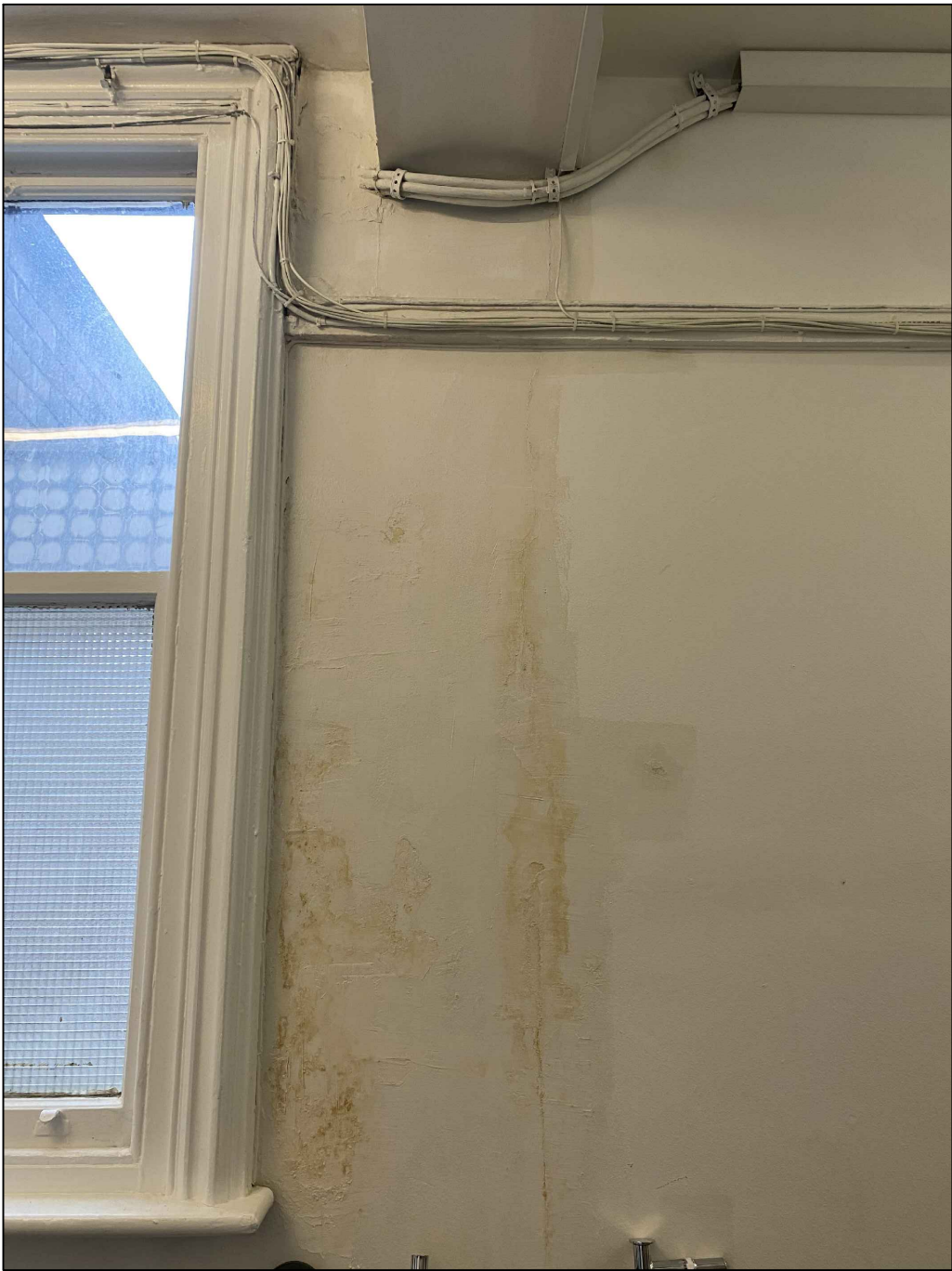
EXISTING ELECTRICAL DISTRIBUTION PHOTO 'A'
