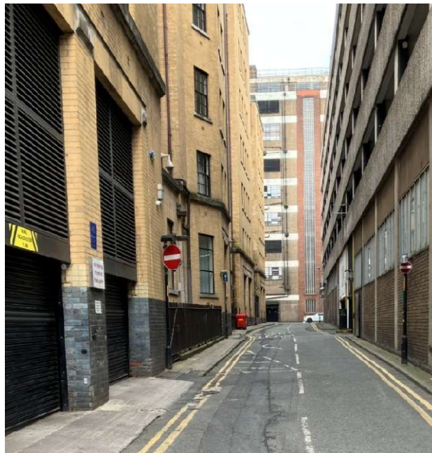
Plate 2: Plain rear façade to Back South Parade
