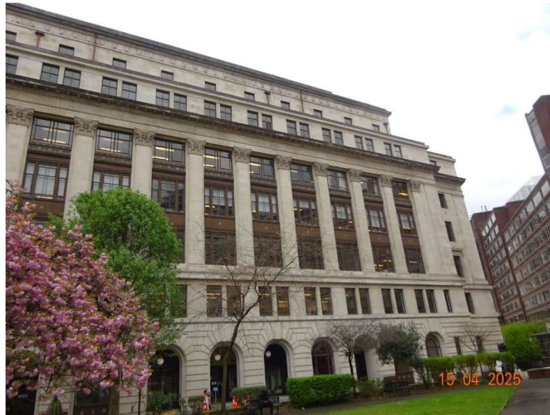
Plate 1: Decorative Portland stone façade to north elevation
