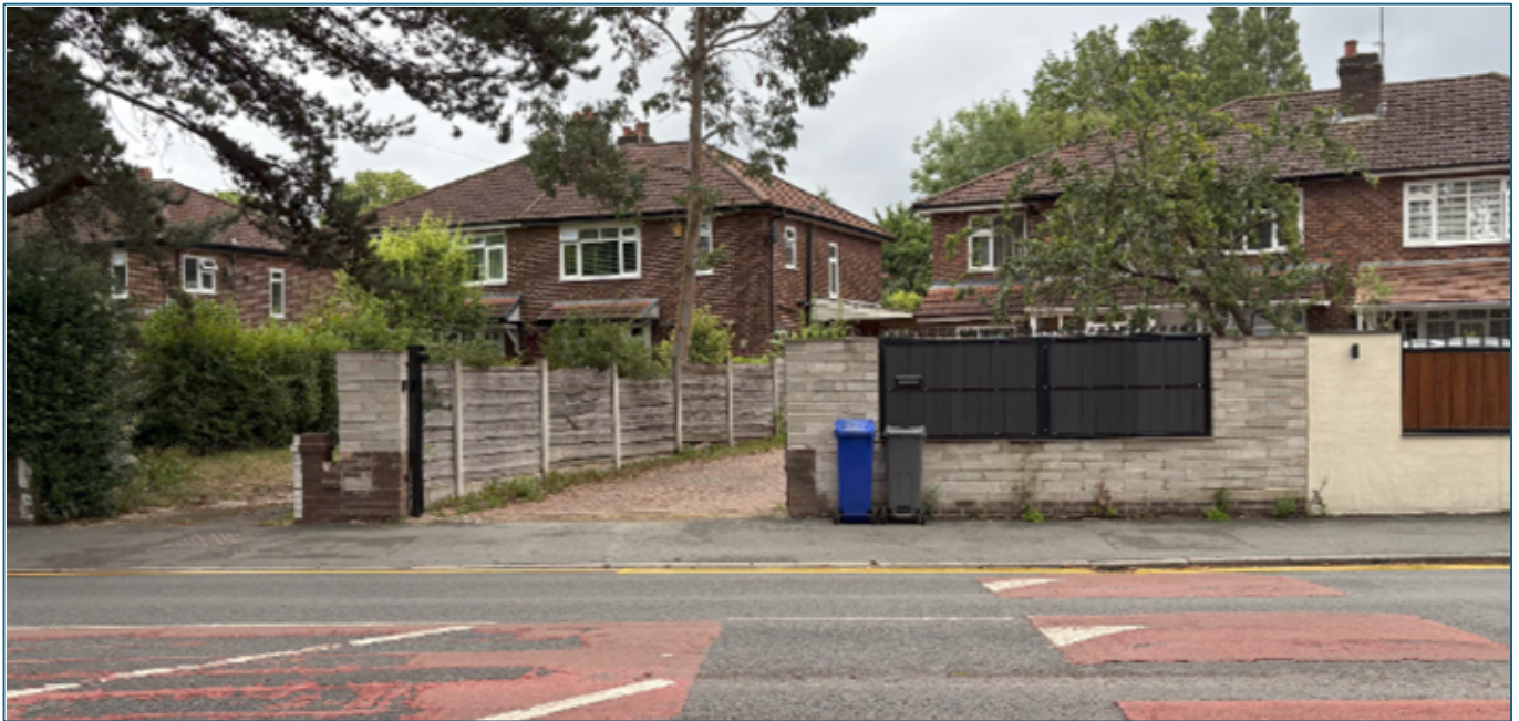
Figure 3. Site visit 02 July 2025
