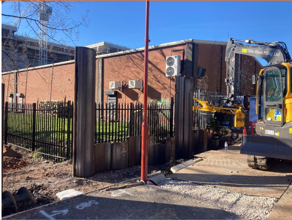
PLATE 03 – INSTALLATION OF LOW PERMEABILITY BARRIER
