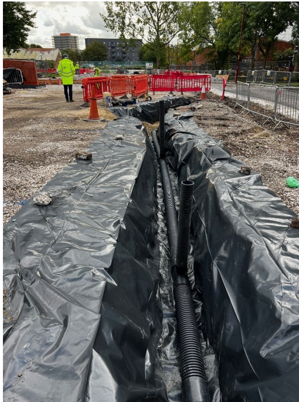
PLATE 07 – INSTALLATION OF POSITIVELY DRAINED HARDSTANDING
