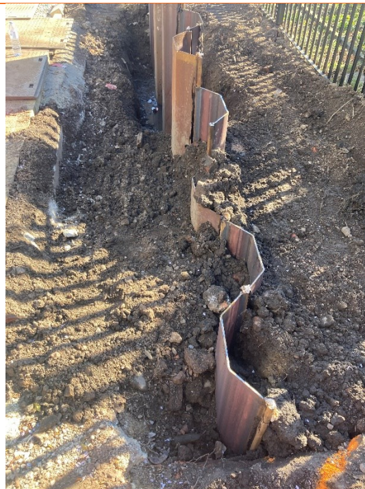
PLATE 04 – INSTALLATION OF LOW PERMEABILITY BARRIER
