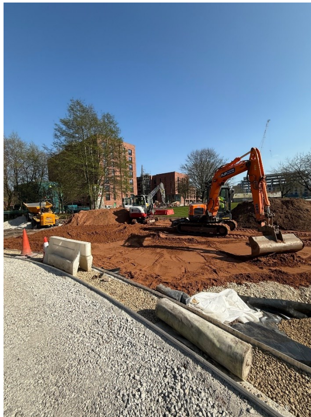
PLATE 10 – INSTALLATION OF POSITIVELY DRAINED HARDSTANDING
