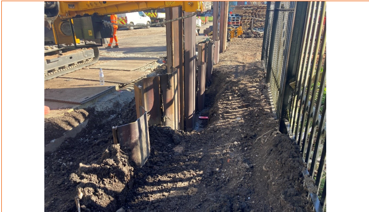
PLATE 05 – INSTALLATION OF LOW PERMEABILITY BARRIER
