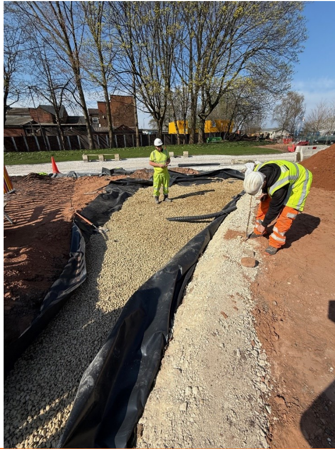
PLATE 10 – INSTALLATION OF POSITIVELY DRAINED HARDSTANDING
