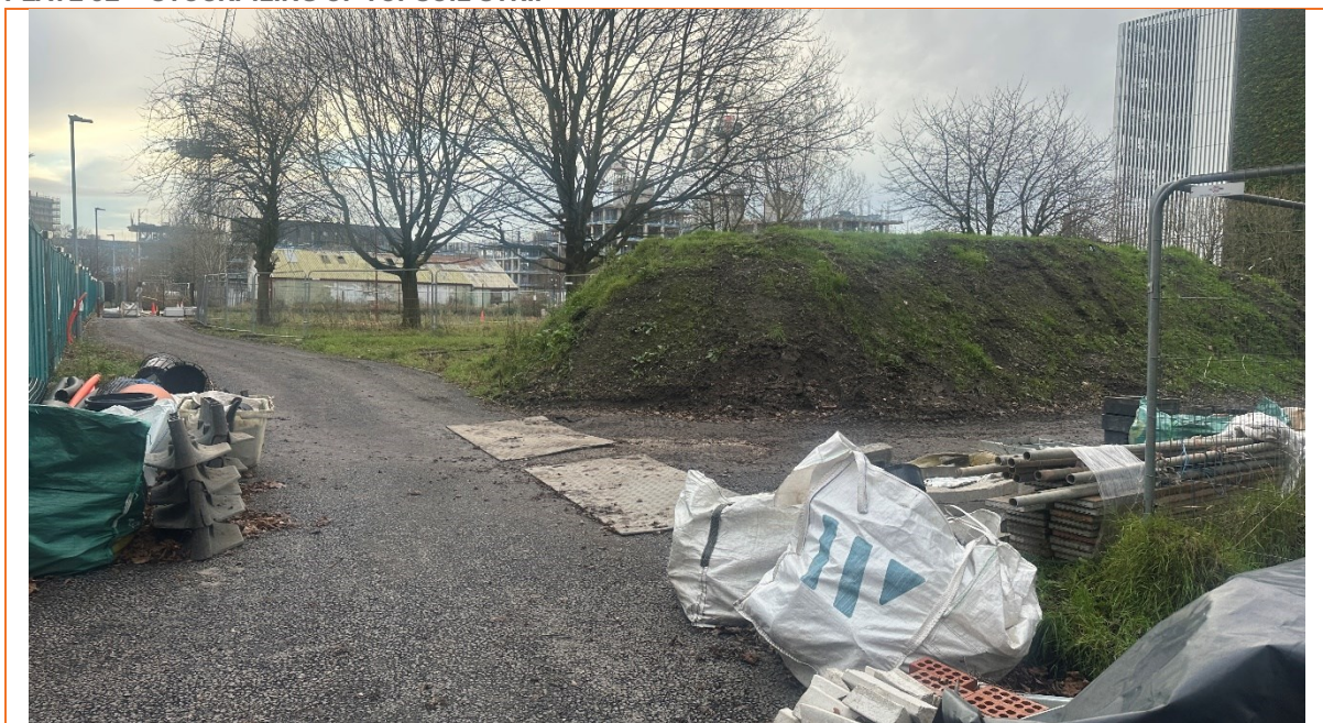
PLATE 02 – STOCKPILING OF TOPSOIL STRIP
