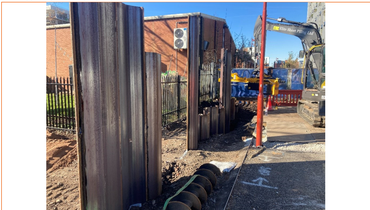
PLATE 06 – INSTALLATION OF LOW PERMEABILITY BARRIER
