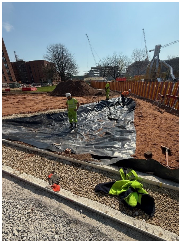
PLATE 08 – INSTALLATION OF POSITIVELY DRAINED HARDSTANDING
