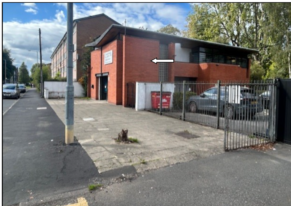
View of application building from car park access
