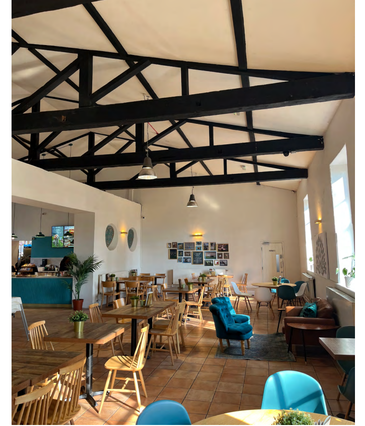
Figure 7 Cafe Interior: Internally the building is contemporary in feel with a mixture of modern wall linings and exposed brickwork, tiled surfaces and exposed services. The original exposed trusses and painted sliding sash windows that remain intact.
