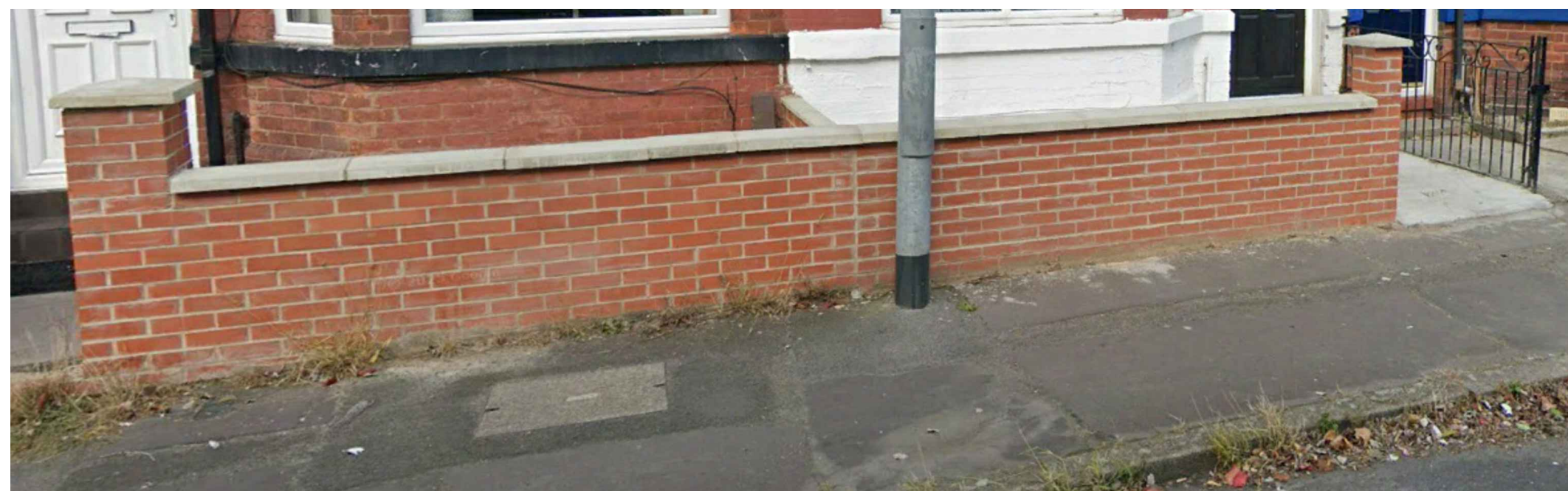
Typical existing boundary treatment to neighboring properties
