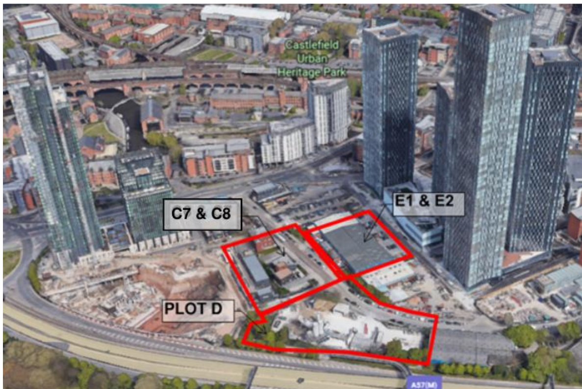
Figure 1 - Google Earth image of the Site Location, 2022
