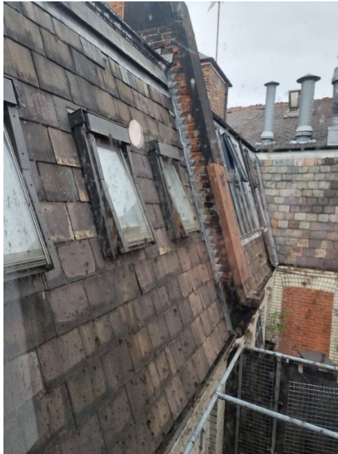
Photograph 8 - View from fourth floor stairwell window looking South East across the mansard serving the fourth floor apartments and down onto the 3.2m high Keyclamp and weldmesh enclosure surrounding the decking. In addition showing 3 No. extract flues serving the adjacent property that were routed with the benefit of bricking up the windows below.
