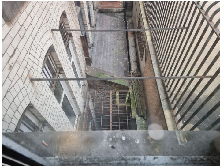
Photograph 6 - View from second floor stairwell window looking down showing white glazed brickwork on the left and 2m high steel railings to the right.
