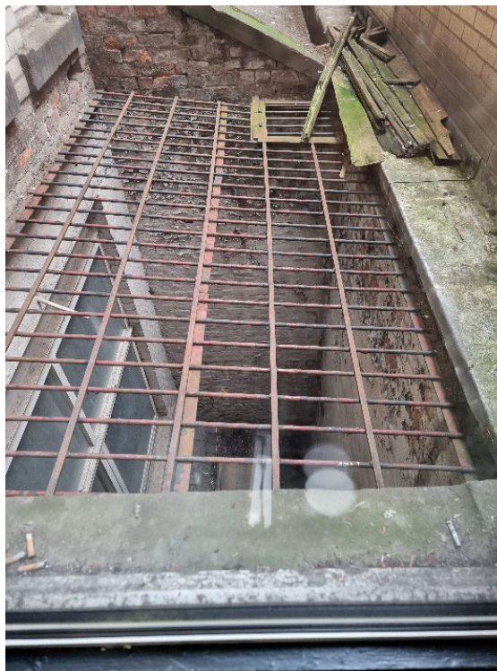
Photograph 3 - View from first floor stairwell window looking down showing security grille above window serving application site.
