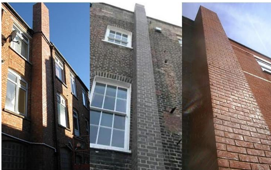
Photograph 9 – Images of similar bespoke GRP flue covers manufactured by GRP Building Products Ltd
