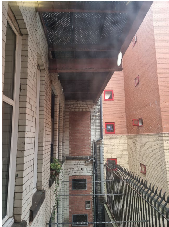
Photograph 2 - View from second floor stairwell window looking East with the decking adjacent to the third floor apartments above. The building to the right being the Your Housing Group apartments “contemporary” design approved by the Council within the conservation area. To the right are windows serving habitable rooms approved by the Council with an area of 0.95m 2 .
