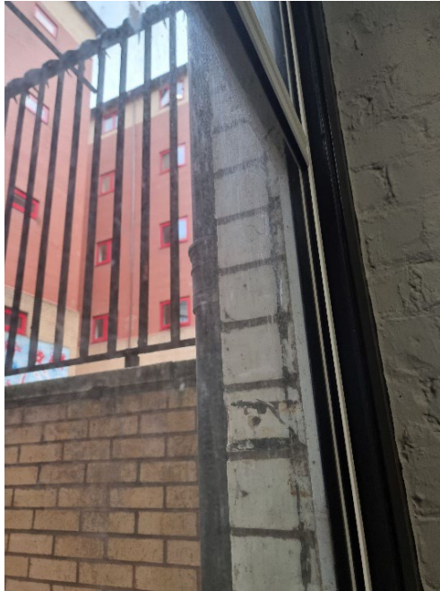
Photograph 10 - View from first floor stairwell window looking South East showing white glazed brickwork to window jamb that will be extended with matching bespoke white glazed brickwork grp enclosure, and existing PVCu rwp that will be re-located to internal corner of rear elevation.
