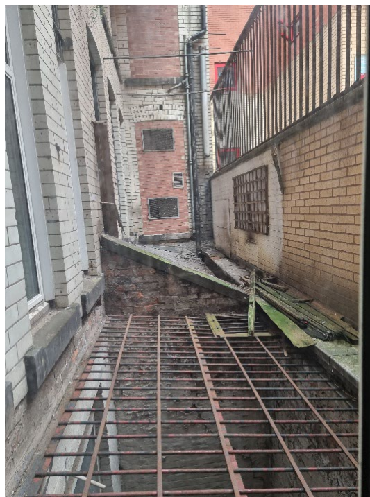
Photograph 1 - View from first floor stairwell window looking East, security grille to lightwell serving the application site below, retaining wall to courtyard serving 117-119 Princess Street to the right, windows to first floor apartments on the left and bricked up former stairwell windows to No.63 Whitworth Street in the distance.
