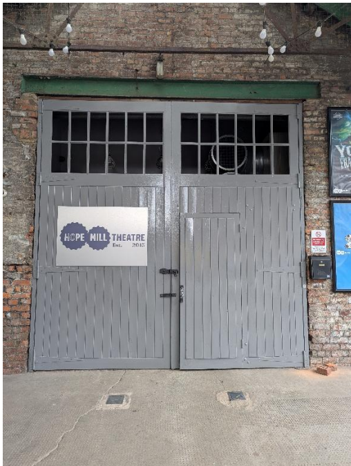
Existing Entrance To Hope Mill Theatre
