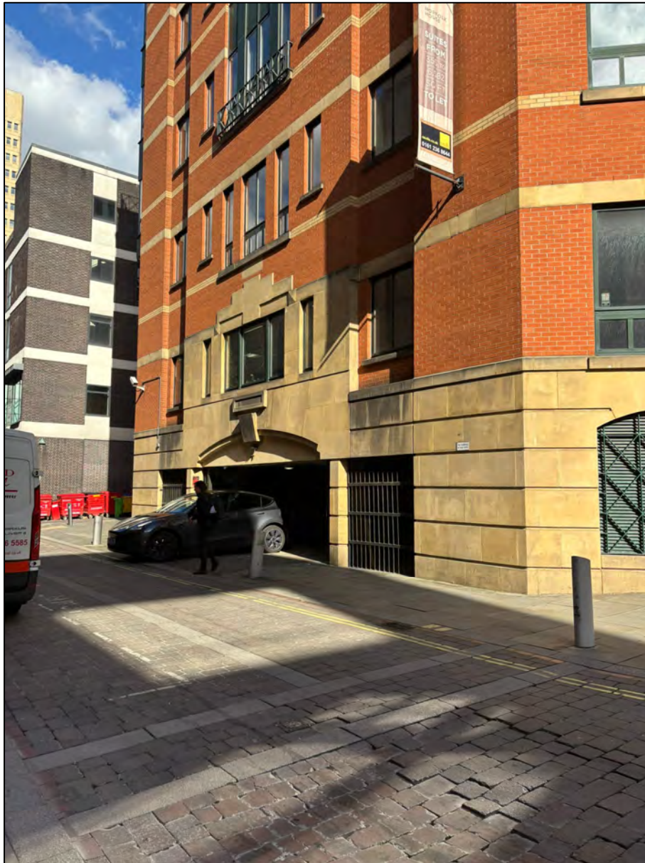
Image 2.4 Existing Vehicular Access
