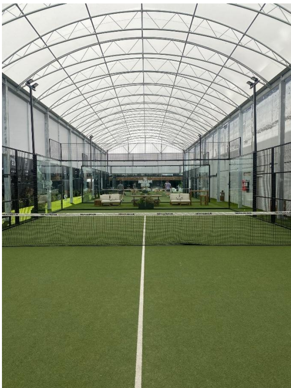
View inside padel courts (canopy roof and walls)
