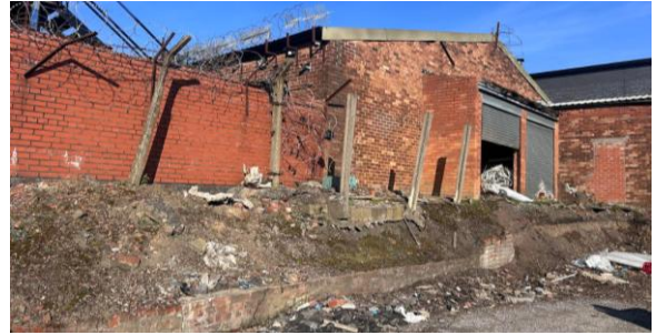
Plate 6 View facing northeast showing retaining wall.
