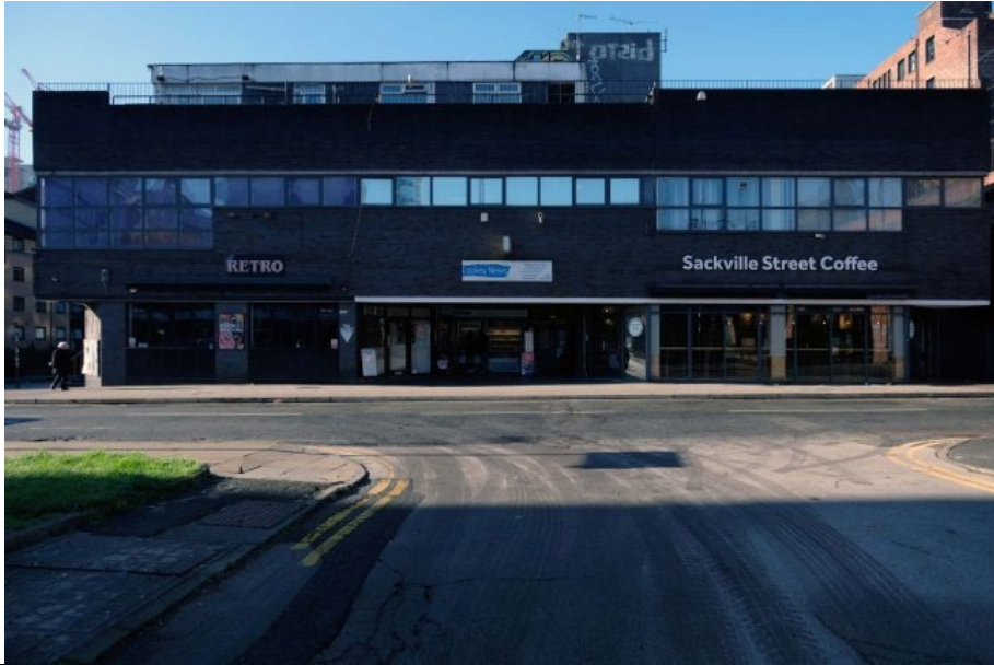
Figure 8: Charles Street car park, east elevation. East block comprises of grey brick in stretcher bond with continual window to upper storey. Ground floor has been extensively altered. Original ‘swinging sporran’ bar now replaced with the ‘retro bar’ and a coffee shop and kiosk also feature.
