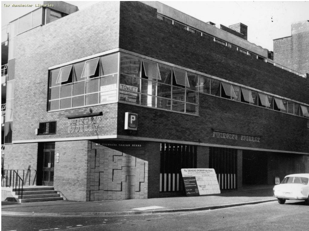
Figure 7: UMIST Car park, Charles Street c.1970s, Manchester. East elevation. Source: Manchester Image Archive.
