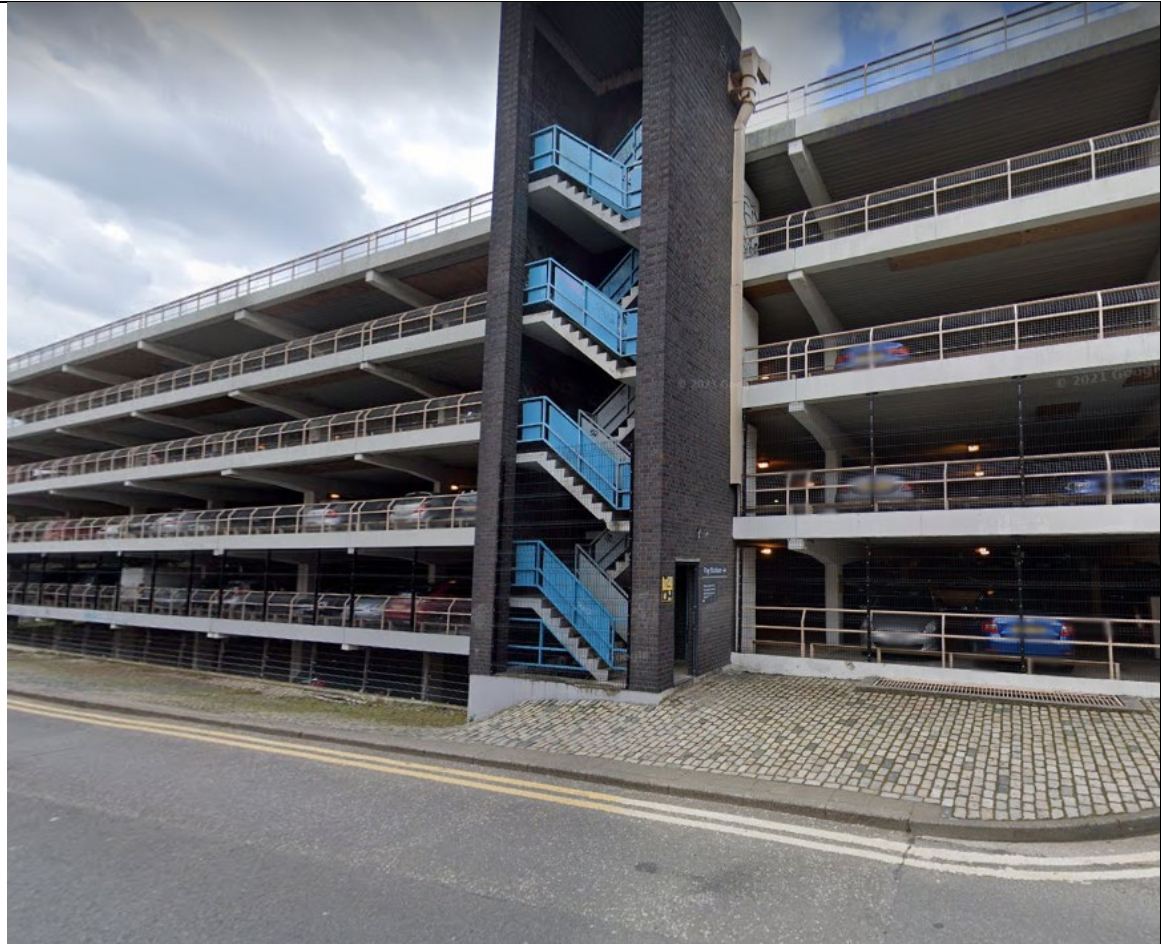
Figure 12: Exposed, multi-storey car park, south elevation. Grey brick external stair. Concrete frame with ribbed ceiling detail and exposed concrete piers. Source: Google street view.
