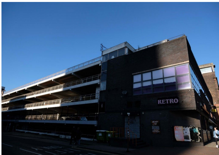
Figure 3: South elevation of the Site, illustrating the open multi-storey car park to the rear.
