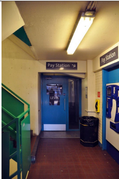
Figure 11: Charles Street Car Park. Internal stair core.
