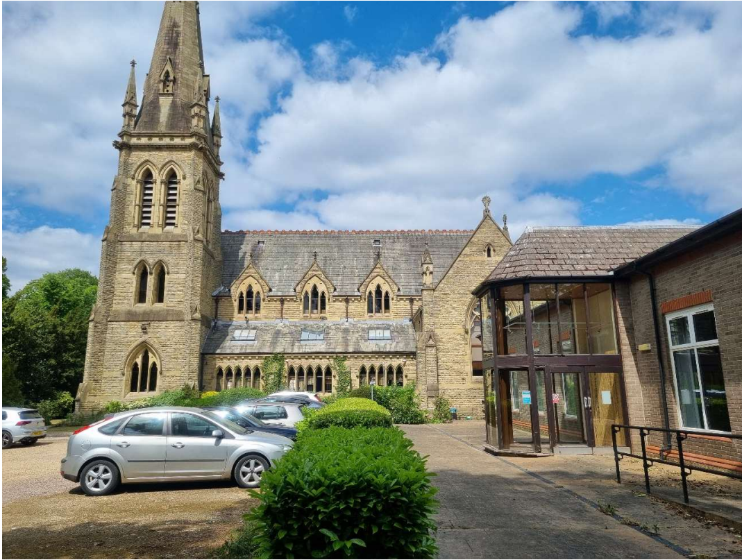
View to South Elevation from southern boundary
