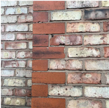
5. PROPOSED BRICKWORK TO MATCH EXISTING Traditional reclaimed light-buff / water-struck brick to match existing for low level wall, with solid red corners and details.
