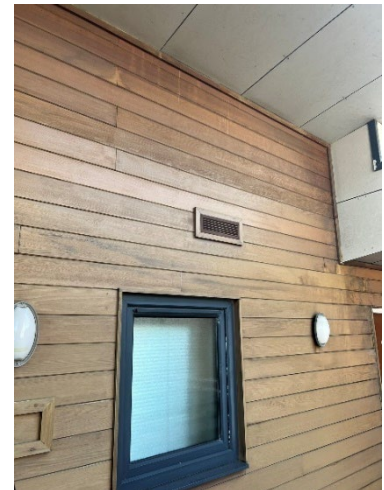
Existing Horizontal Cedar Wood Cladding - Natural
