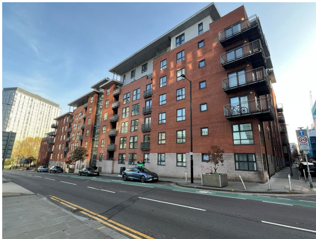
The Linx Building – Angel Street Elevation
