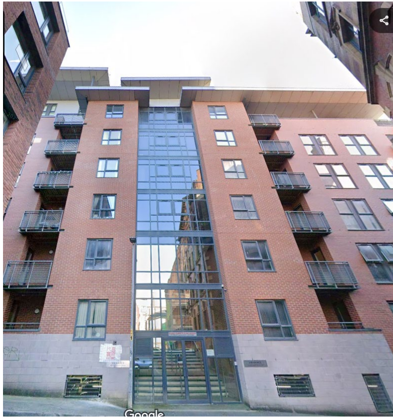
The Linx Building – Ludgate Street Elevation
