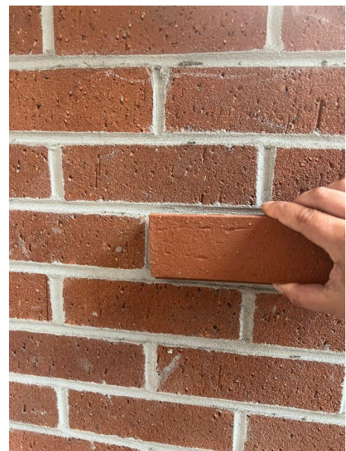
existing facing brick.
