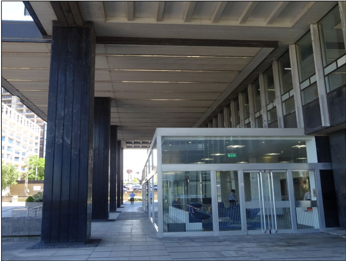
Figure 1. View of Miller Street frontage.
