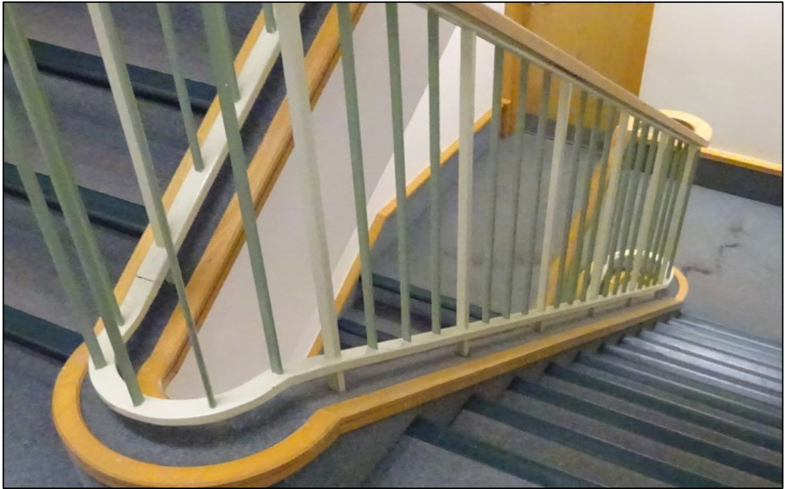
Figure 14 The non-original carpets and handrails to the service stairs on the upper-floors (level 24 and 25).
