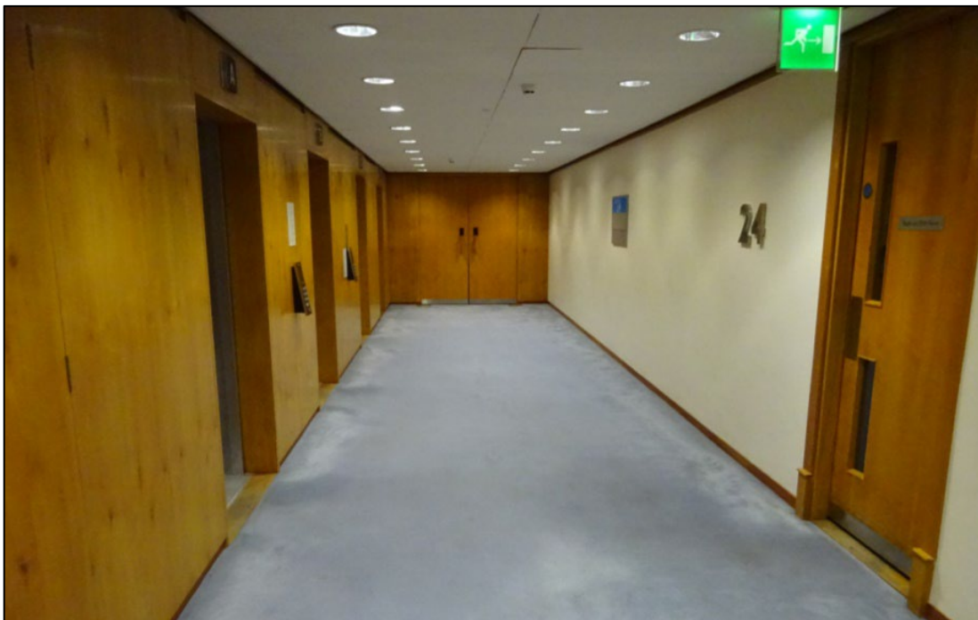
Figure 16. The lift lobby to the 24 th Floor with original doors and panelling to be refurbished.
