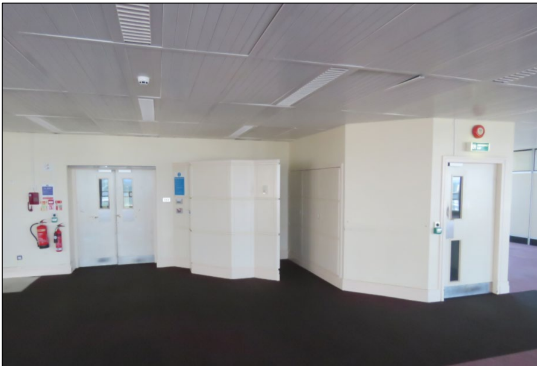
Figure 11. Typical office floor (14 th - floor of the Miller Street tower). The offices will be subject to general refurbishment of the non-original fabric (comprising ceilings, plaster walls, carpets and partitions).
