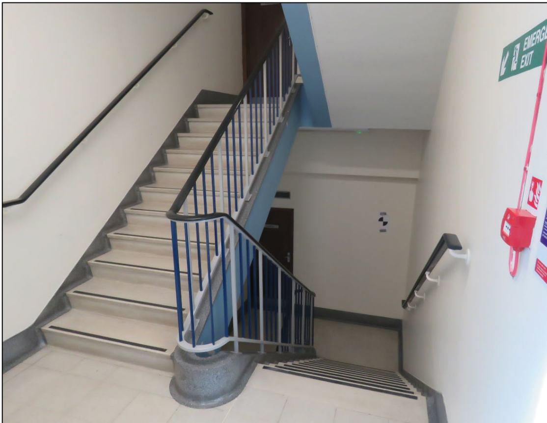
Figure 13. Typical stair core on the office floors with functional terrazzo tiled floors and painted steel balustrades and vinyl handrails in generally good condition.
