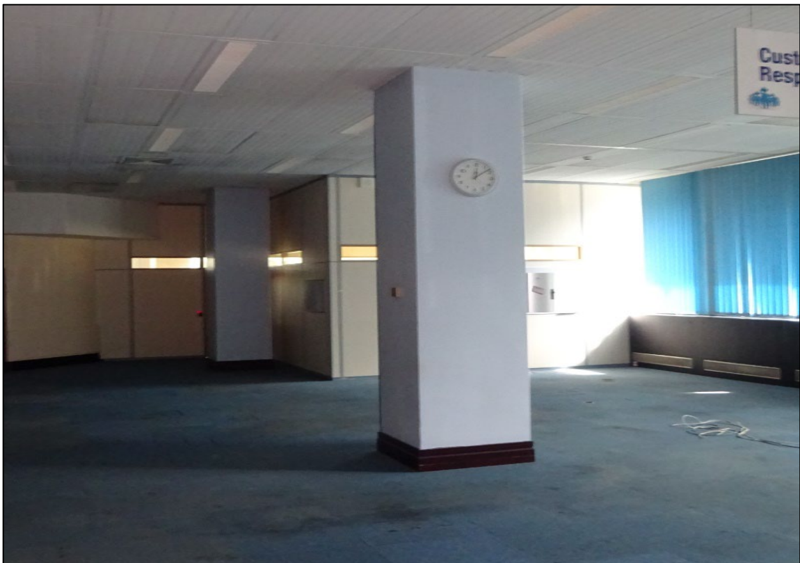
Figure 12. Typical Podium floor office space. All fabric components shown (ceilings, floors, cladding to columns) is non-original and will be made good as necessary.
