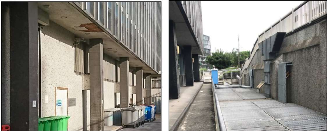
Figure 2. A view of the retained tiles to be cleaned and consolidated (Riga Street light-well).
