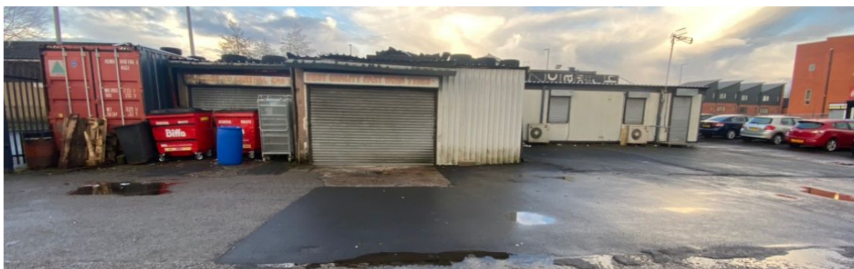
Rear of the structure.
