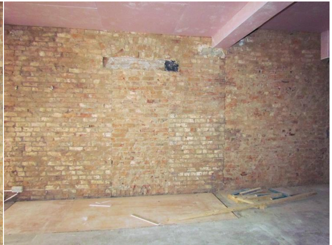
Blocked Doorway and Altered Floor
