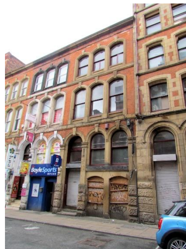
Front Elevation of No. 46
