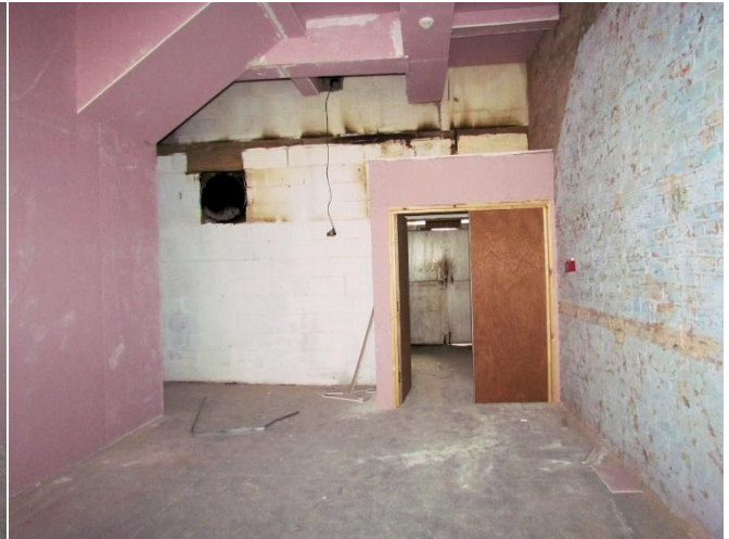
Block Wall Enclosing Staircase
