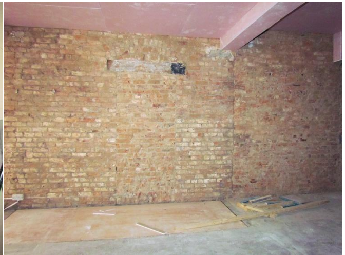
Blocked Doorway and Altered Floor
