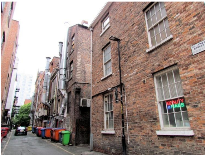
View North-east Along St James Street Showing Former Warehouses on the South- east Side
