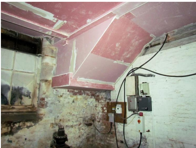
Steps to Ground Floor Above
