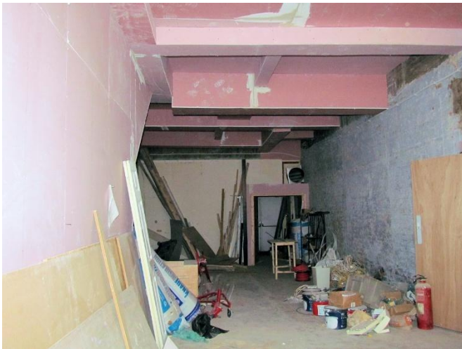
Ground Floor, Looking North-west
