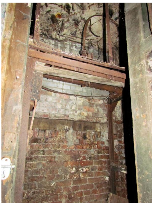
Upper Part of Service Lift Shaft
