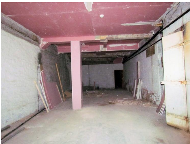
Basement, Looking North-west
