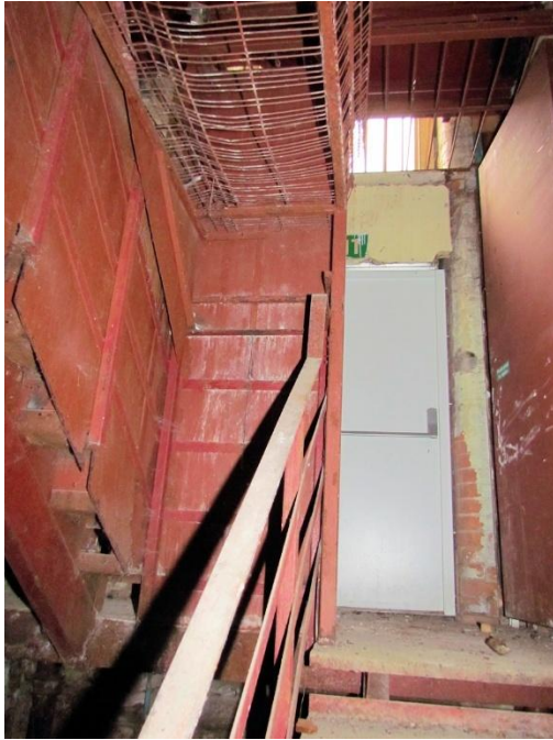
Late 20 th Century Staircase at Rear
