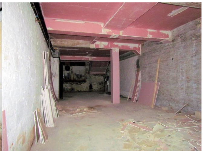
Basement, Looking South-east
