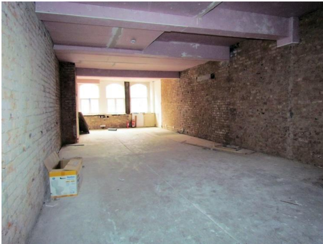
2 nd Floor, Looking South-east
