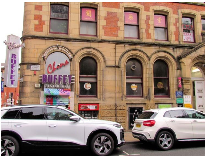
North-east Elevation of 44 Faulkner Street
