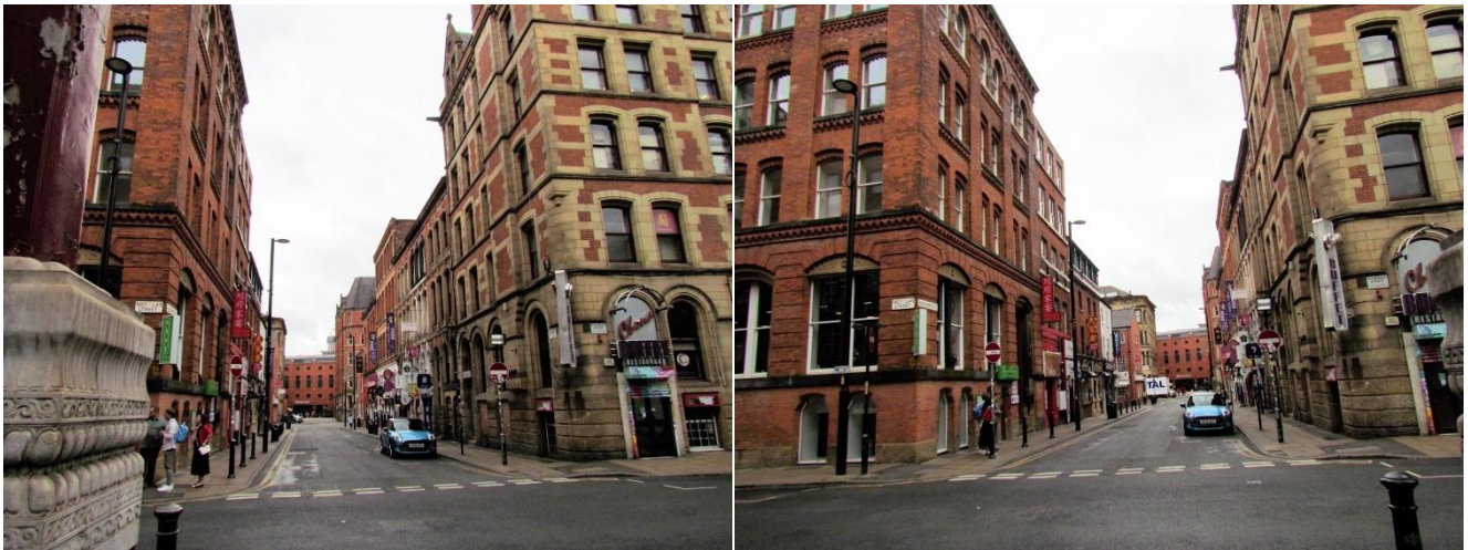
View South-west Along Faulkner Street, Showing Former Warehouses on the North- west Side
