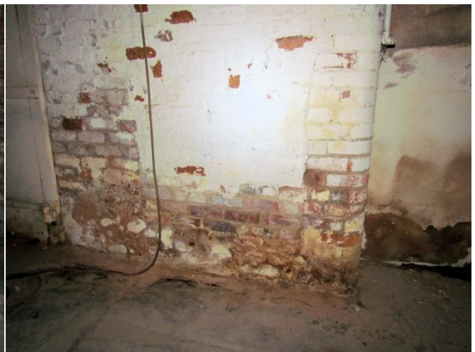
Infilled Opening to Chimney Breast
