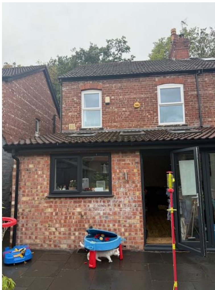
Rear elevation of the application site
