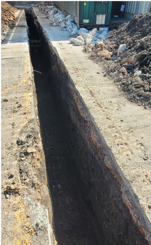
Photograph 1 – Trial Pit Viewing East
