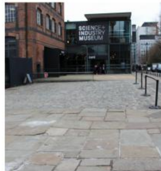
Poorly accessible route from Lower Byrom Street
