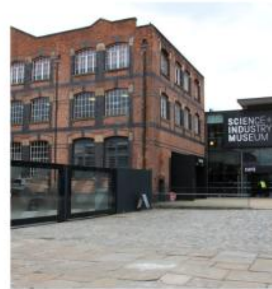
View of the gates and entrance
