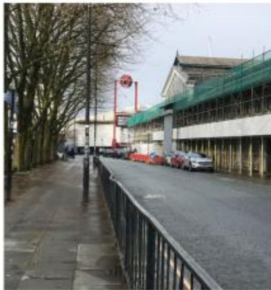
Approach to the Site from Liverpool Road, East
