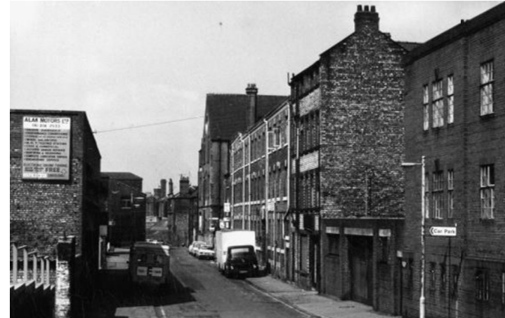
VIEW WESTWARDS DOWN LITTLE PETER ST. 1973.
