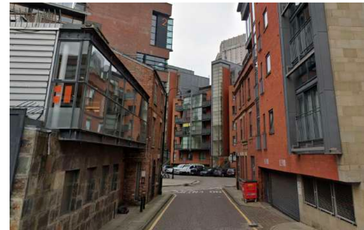
1. 2-4 LITTLE PETER STREET (LEFT), NEIGHBOURING SITE.
