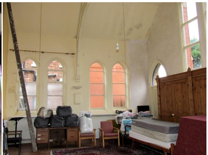
North Part of Interior
