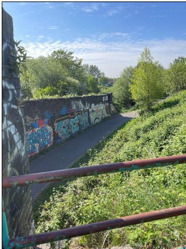
Photo 3: View looking north down onto Fallowfield Loop from the bridge on site.
