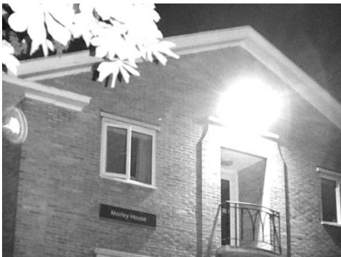
Photograph 15: Morely House - B26B
