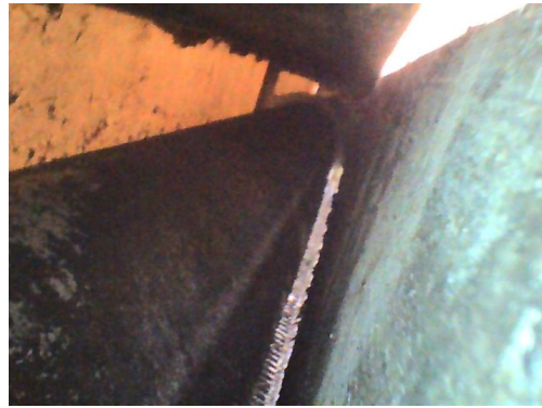
Photograph 18: Endoscopic view of behind fascia board
