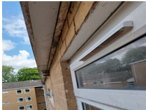
Photograph 5: MEWP inspection of B21
