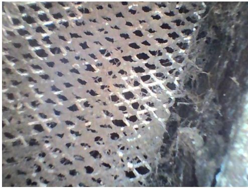
Photograph 17: Endoscope view of metal meshing present on B15, 16, 17, 20 and B21.
