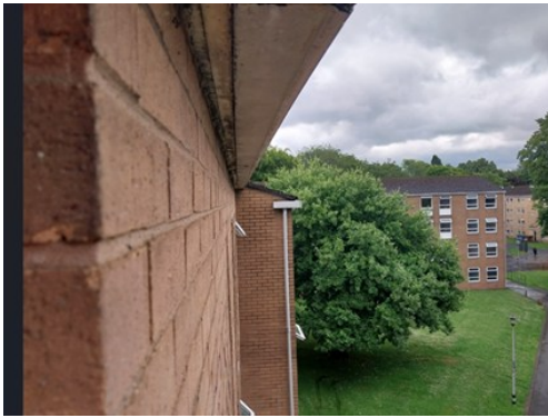
Photograph 9: MEWP inspection of B17
