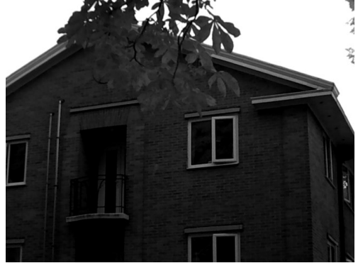
Photograph 12: Lindsay House - B25C
