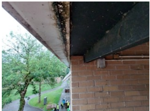
Photograph 8: MEWP inspection of B20
