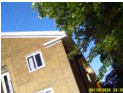
Photograph 7: Spencer House - B24B
