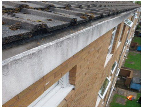
Photograph 2: Slate tile roofing present on all buildings surveyed.
