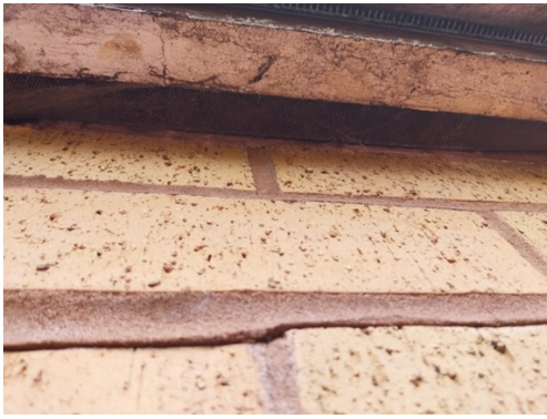
Photograph 1: Metal mesh present on all buildings surveyed
