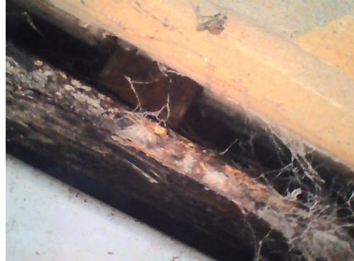
Photograph 20: Endoscopic view of behind fascia board
