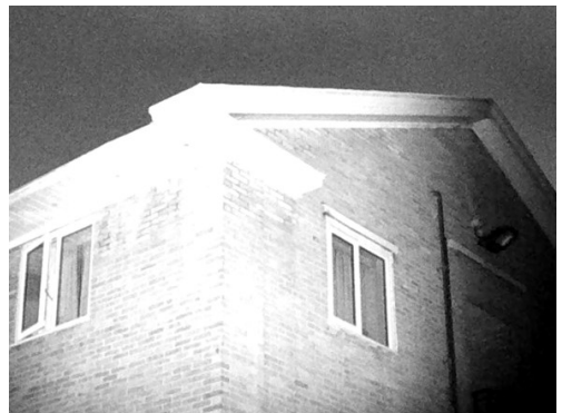
Photograph 16: Morely House - B26C
