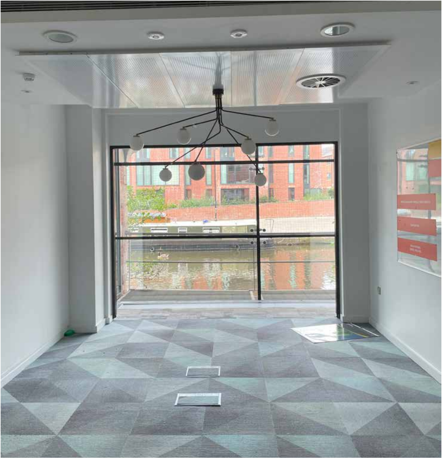
EX.01.09 Meeting room - Ventilation grilles, floor boxes, signage, raised access flooring, carpet tiles Dem.01 / 06 / 11 / 13 / 16 / 27 / 28 / 29 / 33
