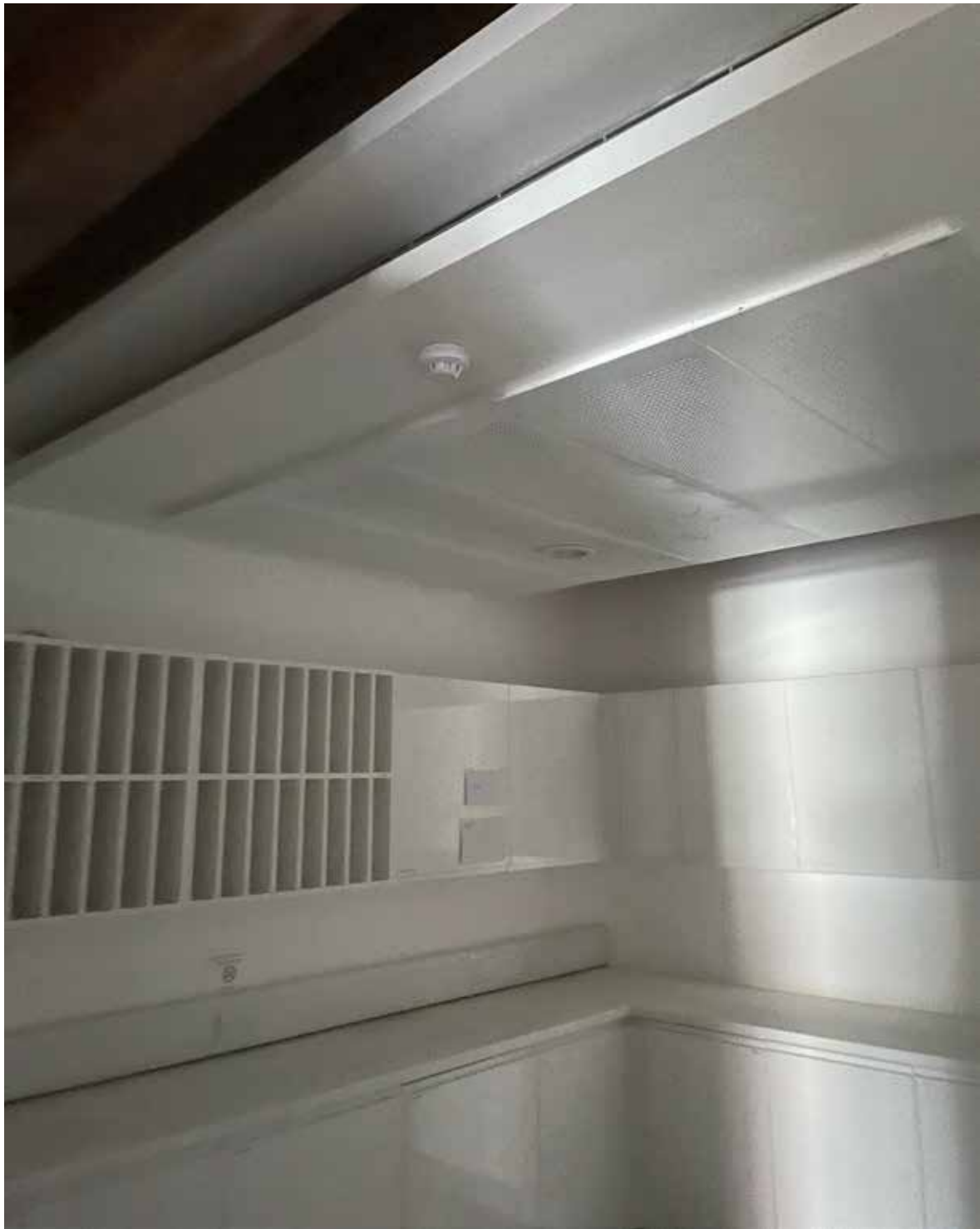
EX.01.03 Post room - Worktops, bespoke joinery, ceiling fixtures Dem.02 / 07 / 08 / 27
