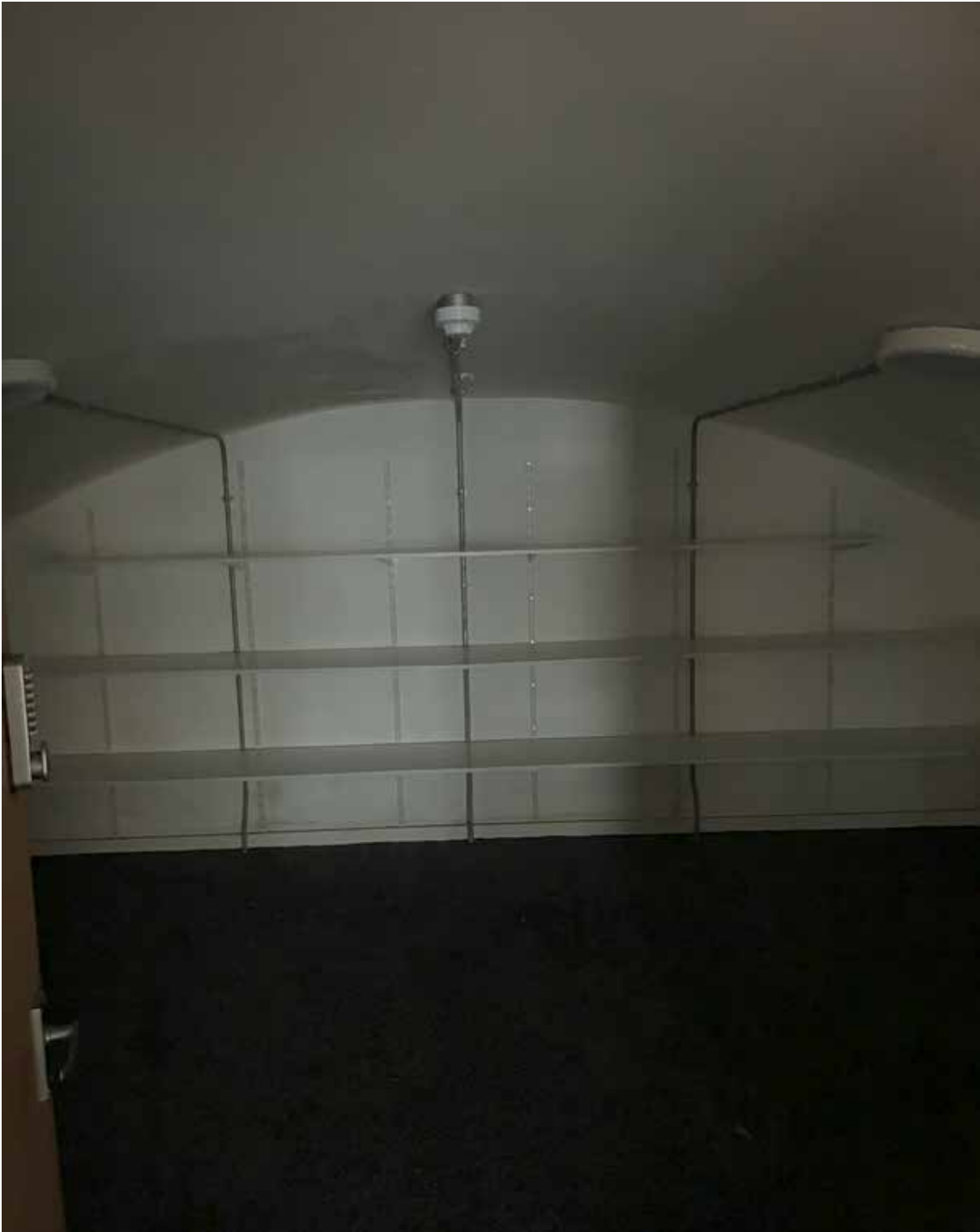
EX.01.14 Store - Sub-dividing partition, floor finishes Dem.01 / 34
