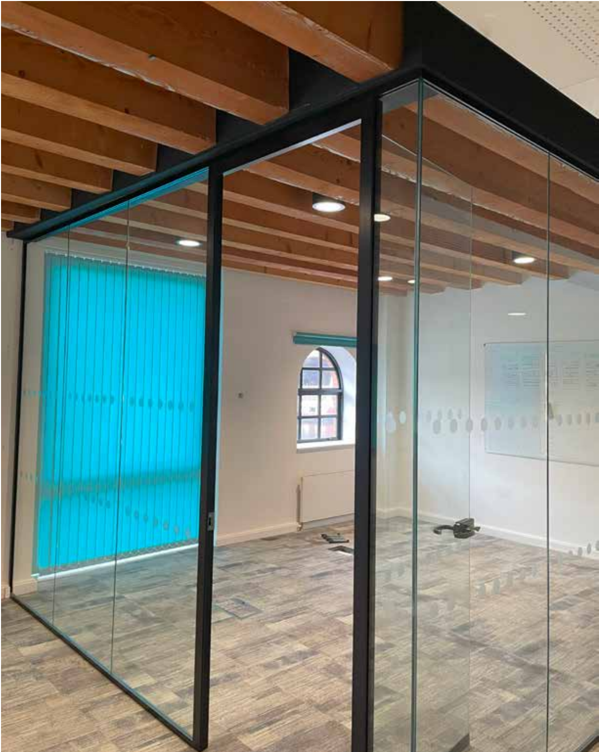
EX.02.12 Meeting room - Glazed partition screen, floor boxes, ventilation, wall sockets Dem.36 / 39 / 41 / 42 / 46 / 47 / 57 / 64 / 66 / 67
