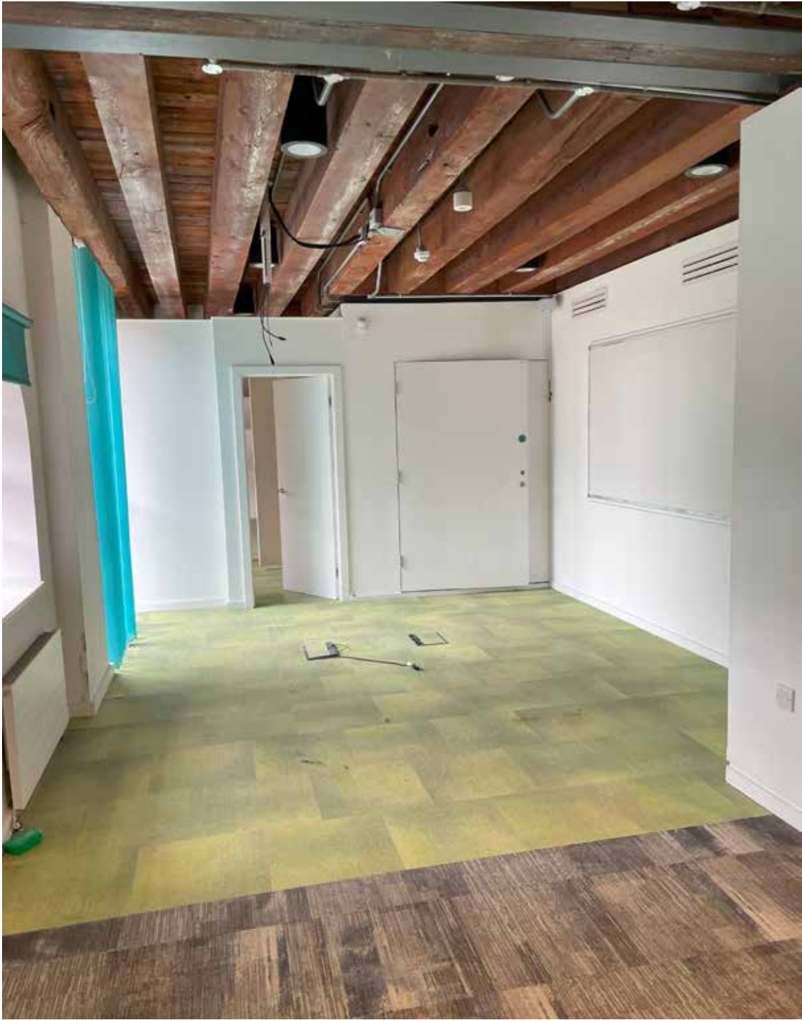
EX.02.04 Office - Carpet tiles, floor boxes, window blinds, riser doors, ventilation grilles Dem.36 / 39 / 41 / 46 / 47 / 53 / 57 / 64 / 66
