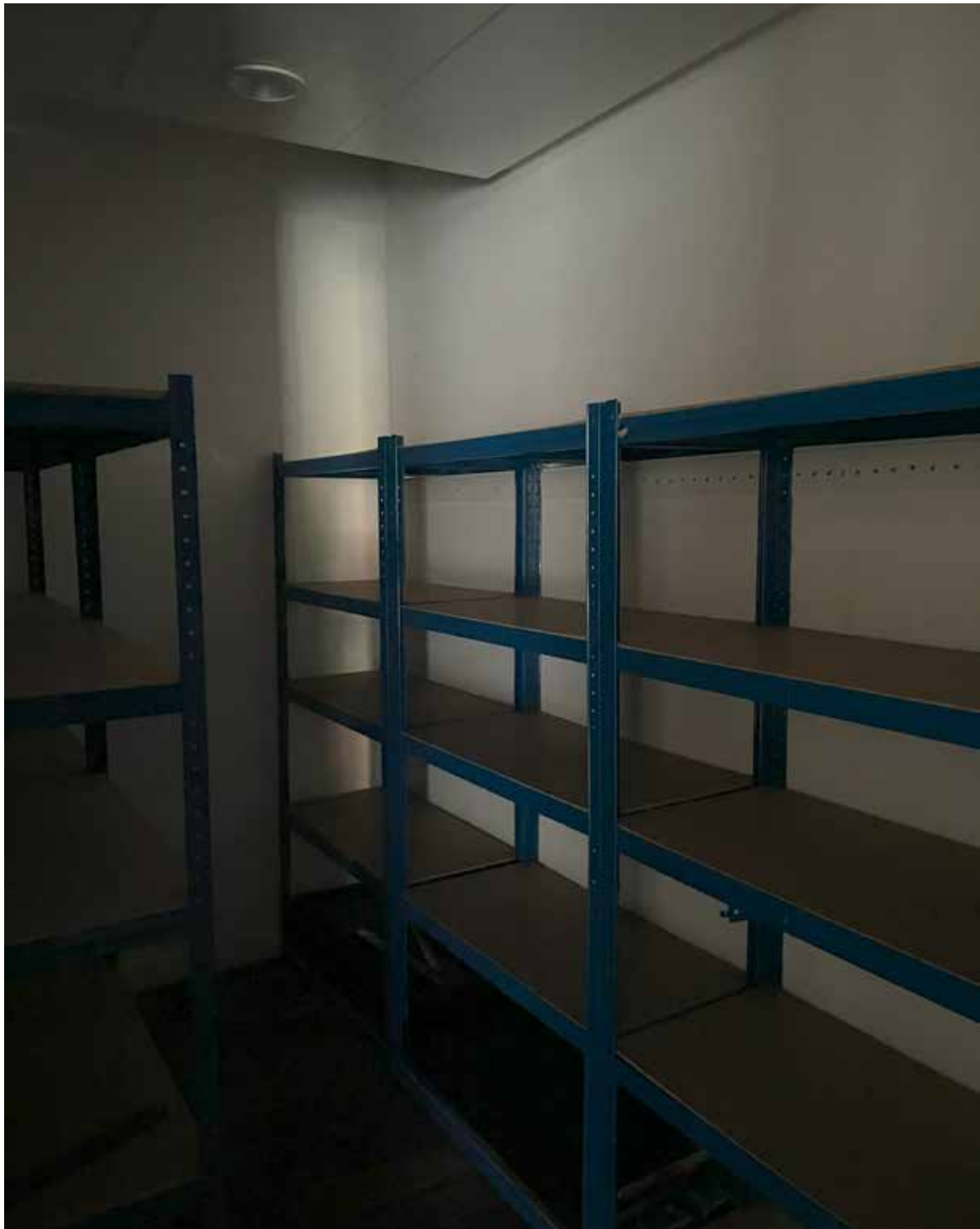
EX.01.22 Store - Existing partitions and room temperature controllers Dem.01 / 07 / 27
