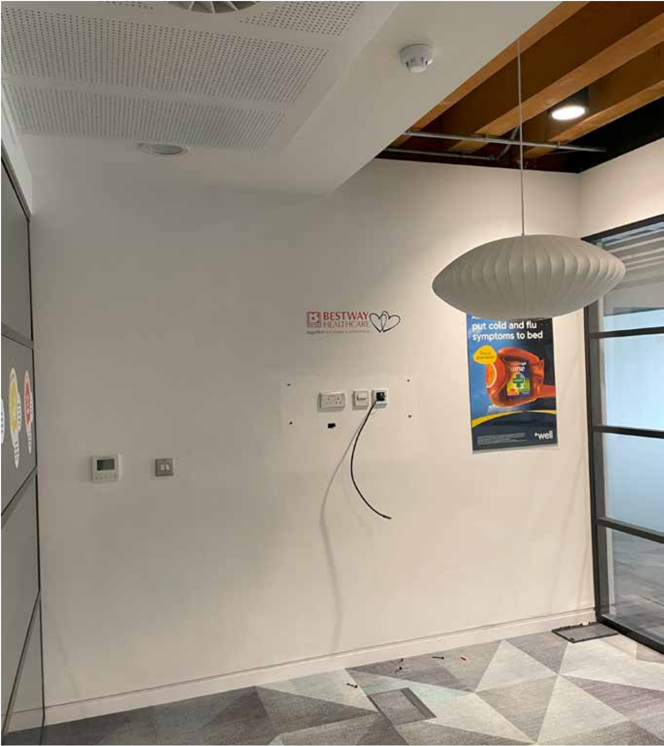
EX.01.13 Meeting room - Glazed partition screens, raised access floor, wall mounted power supply Dem.01 / 06 / 07 / 08 / 11 / 13 / 16 / 23 / 27 / 28
