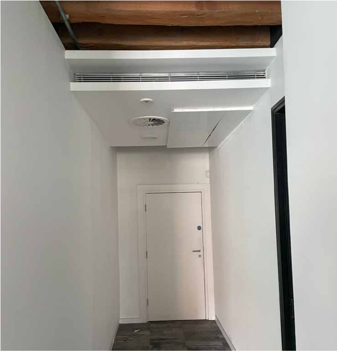
EX.01.22 Store - Existing partitions, ceilings, finishes, room temperature controllers Dem.01 / 28
