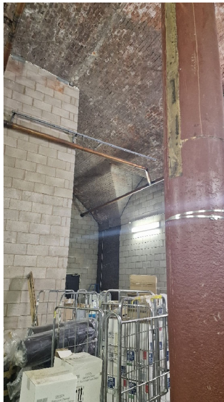
Brick Piers and Vaulted Arches
