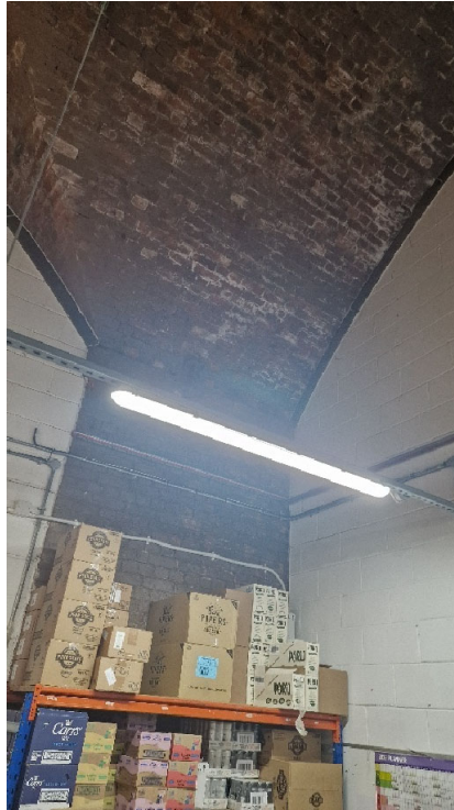
Brick Vaulted Arches
