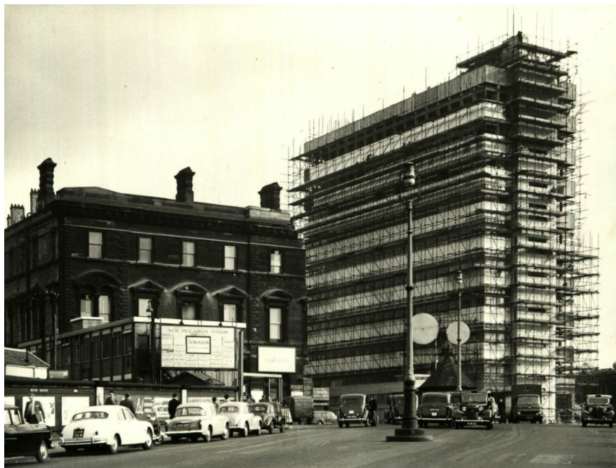
Construction of New Concourse and Office Tower – Photograph from Network Rail Archive
