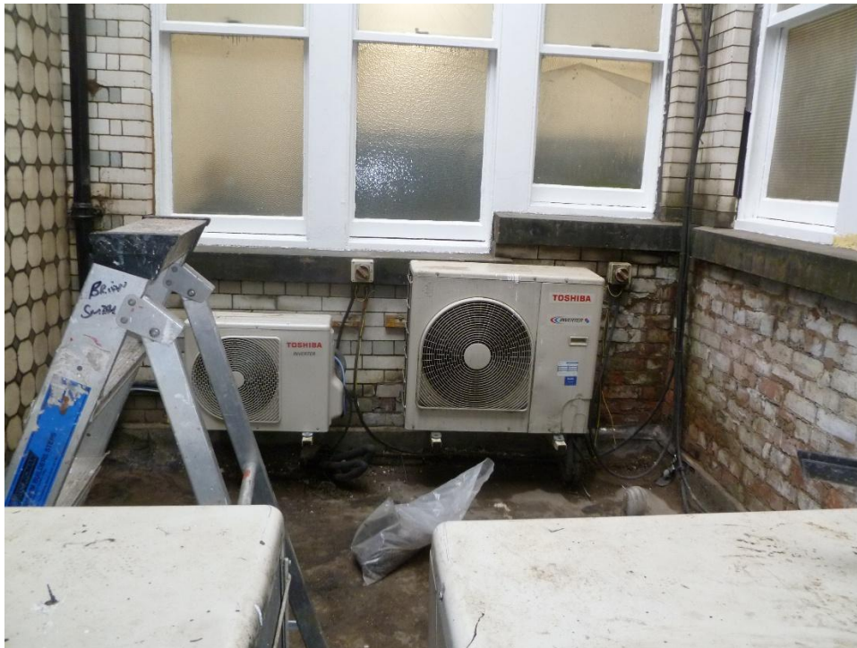
Figure 7.2 Lightwell at December 2025, Source: PBA Site Photograph (Note: the unit to the r/h side foreground has been removed since this image was taken and a new roof installed).
