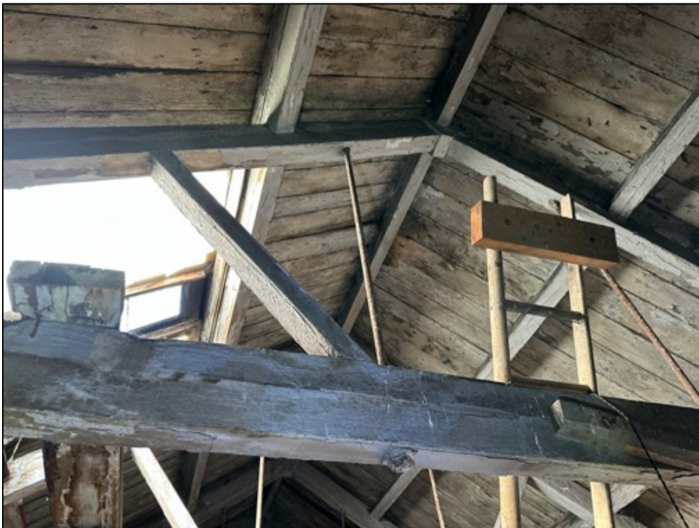
Photograph 12; This section of the roof features some skylight windows within the roof.
