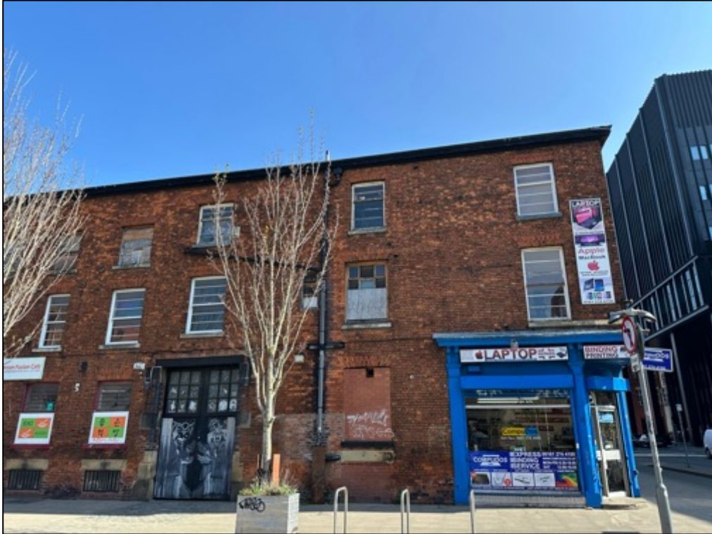
Photograph 3; Another external view of the western face. As mentioned, the building is still in active use at ground level for vendors.
