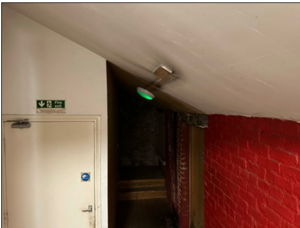
Photograph 13; Many of the rooms on the upper floors featured vaulted ceilings.
