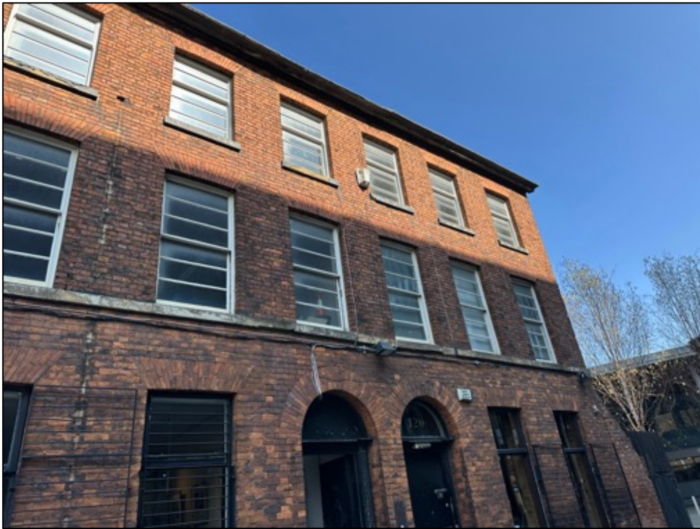
Photograph 5; A front view of the subject building.
