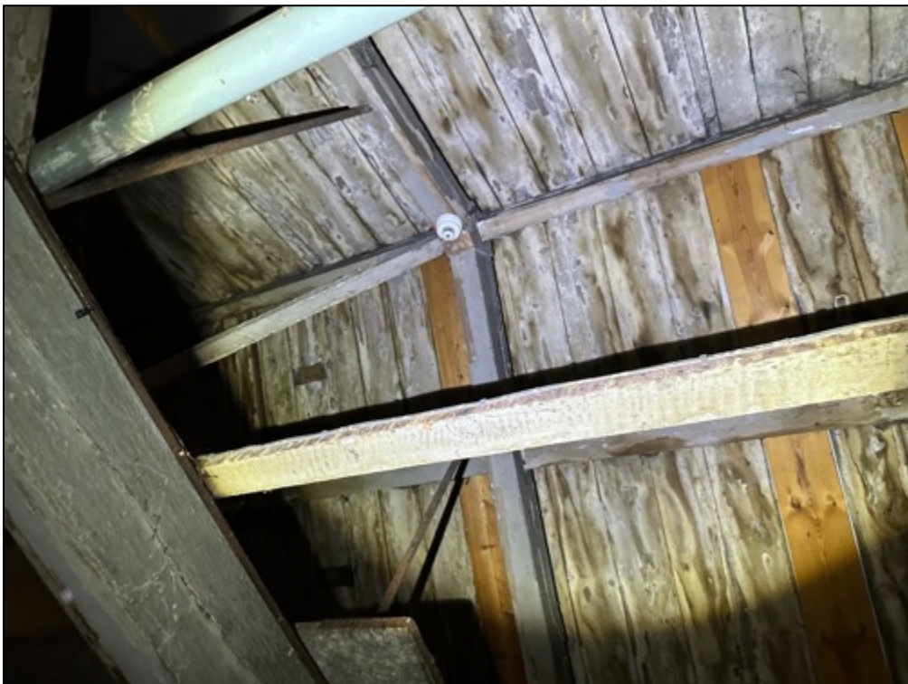
Photograph 10; A view of another section of the internal loft space, showing the internal roof structure. This section consists of wooden boarding supporting the external roof, along with wooden purlins and rafters providing additional structural support.
