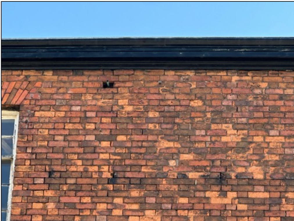
Photograph 4; A closer view of the soffit and fascia structuring beneath the roof. Brickwork is in fair condition, though with some prominent gaps in the mortar.
