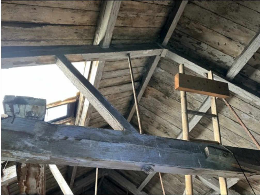
Photograph 11; A view of the open internal section, which is seemingly an unfinished work area. The roof space again, comprises wooden boarding beneath the roof tiles with wooden purlins and rafters supporting.
