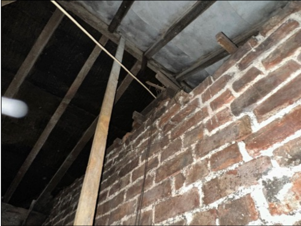
Photograph 9; A section of the internal wall within the roof space was observed to be in good condition.
