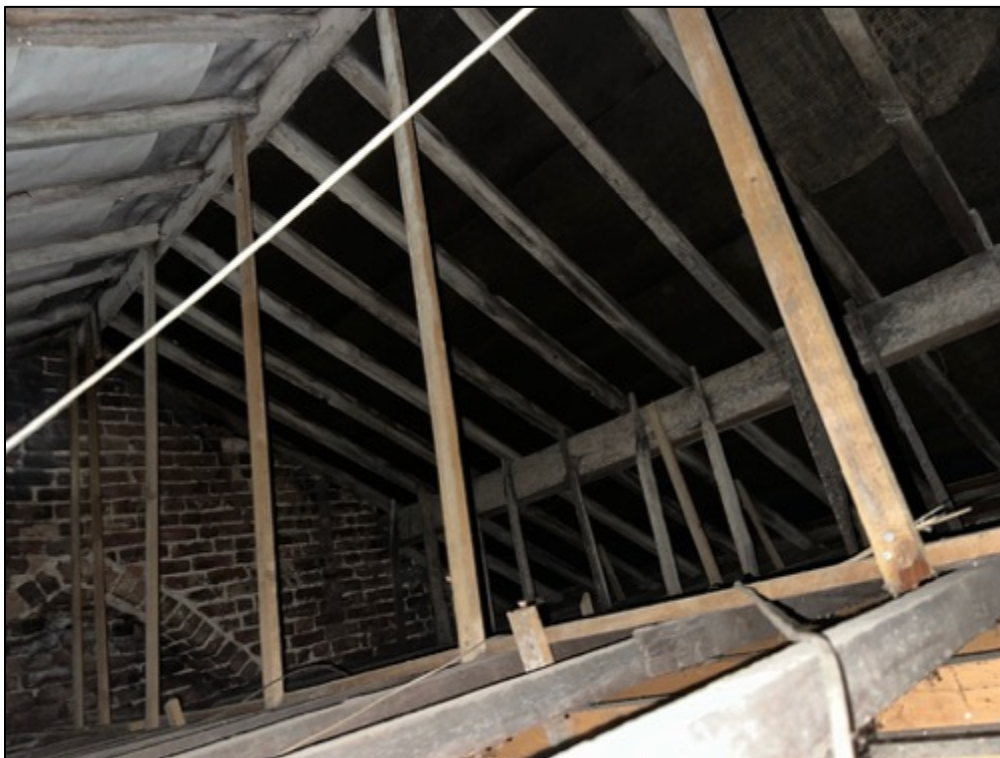
Photograph 7; A view into one section of the internal roof space was obtained through a loft hatch; however, due to the hatch's small size, the inspection was limited to observations from the opening. As a result, the floor of this roof section could not be fully assessed for signs of bat activity.
