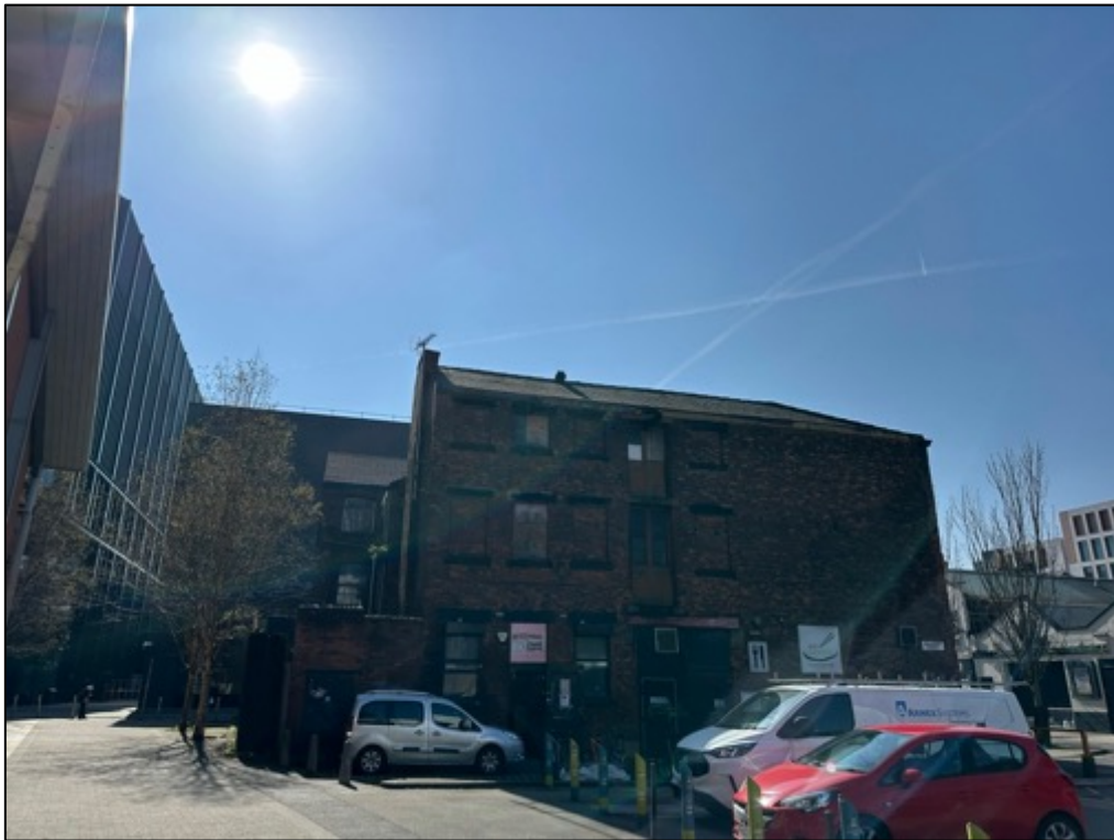
Photograph 1; An external view of the northern face of the building. Majority of external windows have been boarded or bricked over.
