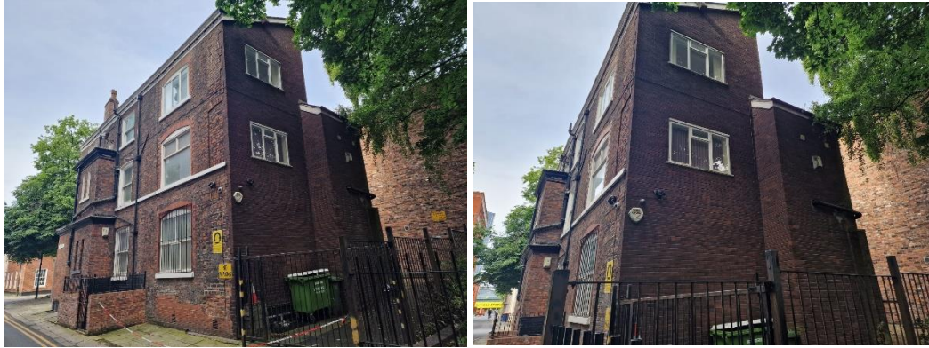
Figure 4.3: Side and Rear Elevation to 8 and 8a St John Street (June 2024)
