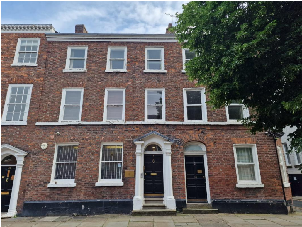
Figure 4.1: 8 and 8a St John Street (June 2024)
