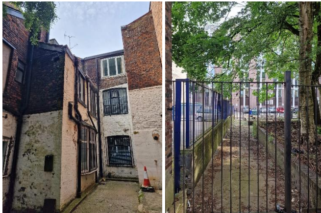
Figure 4.10: Courtyard to Nos 8 and 8a St John Street (June 2024)
