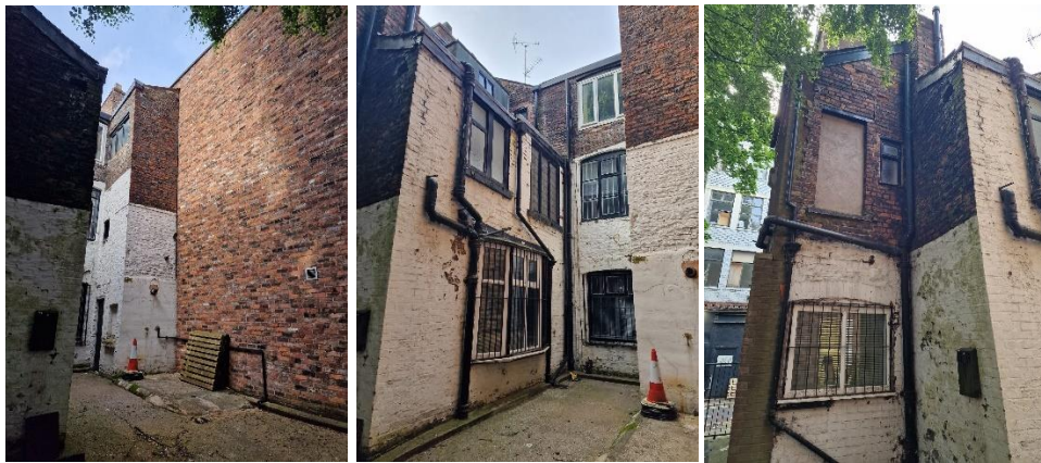
Figure 4.4: Rear Elevation to 8 and 8a St John Street (June 2024)
