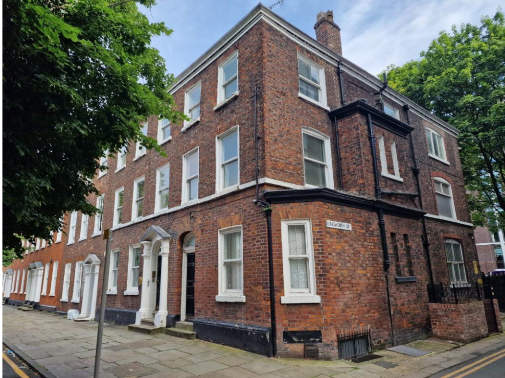
Figure 4.2: 8 and 8a St John Street (June 2024)
