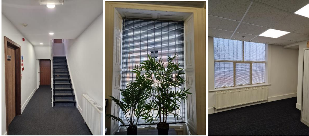
Figure 4.6: Ground Floor to No 8 St John Street (June 2024)
