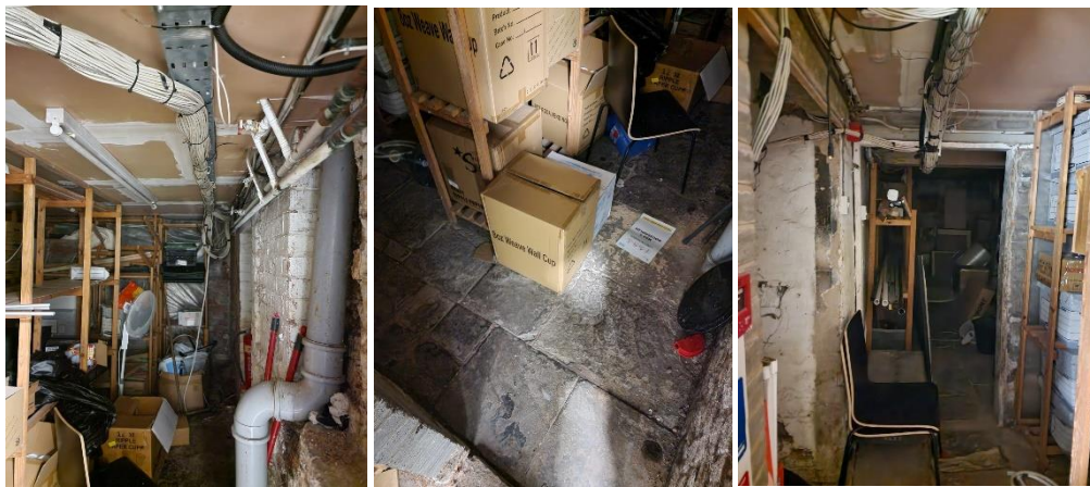
Figure 4.5: Basement to No 8 St John Street (June 2024)
