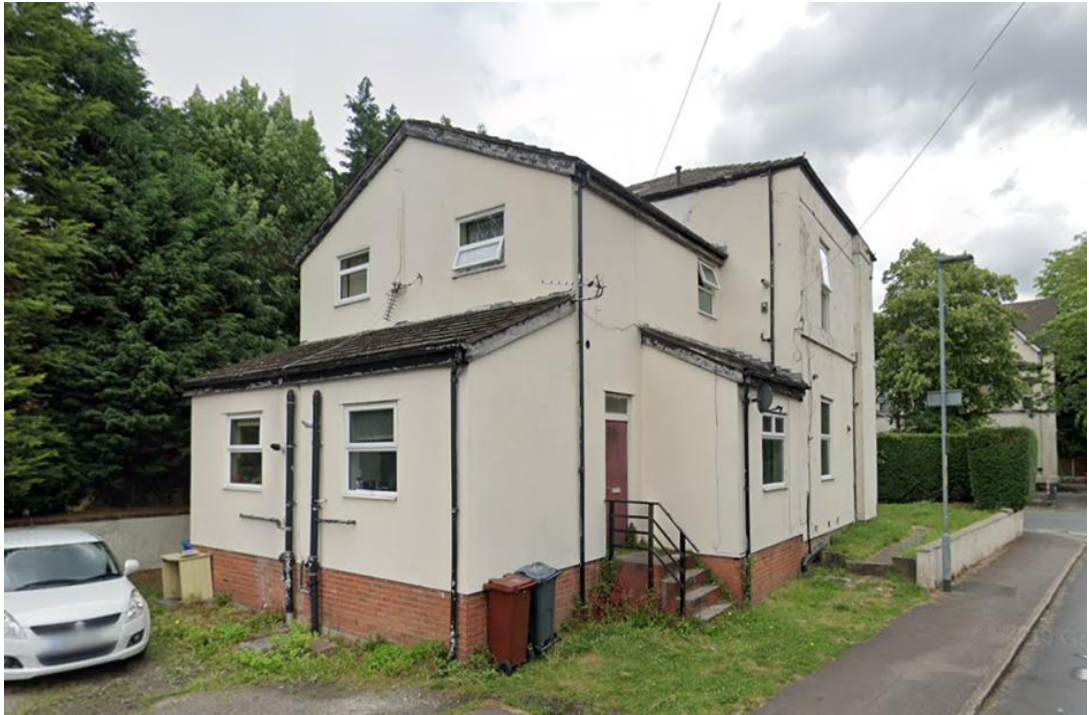
Image 3 – Streetview of rear elevation showing the non-original extensions.
