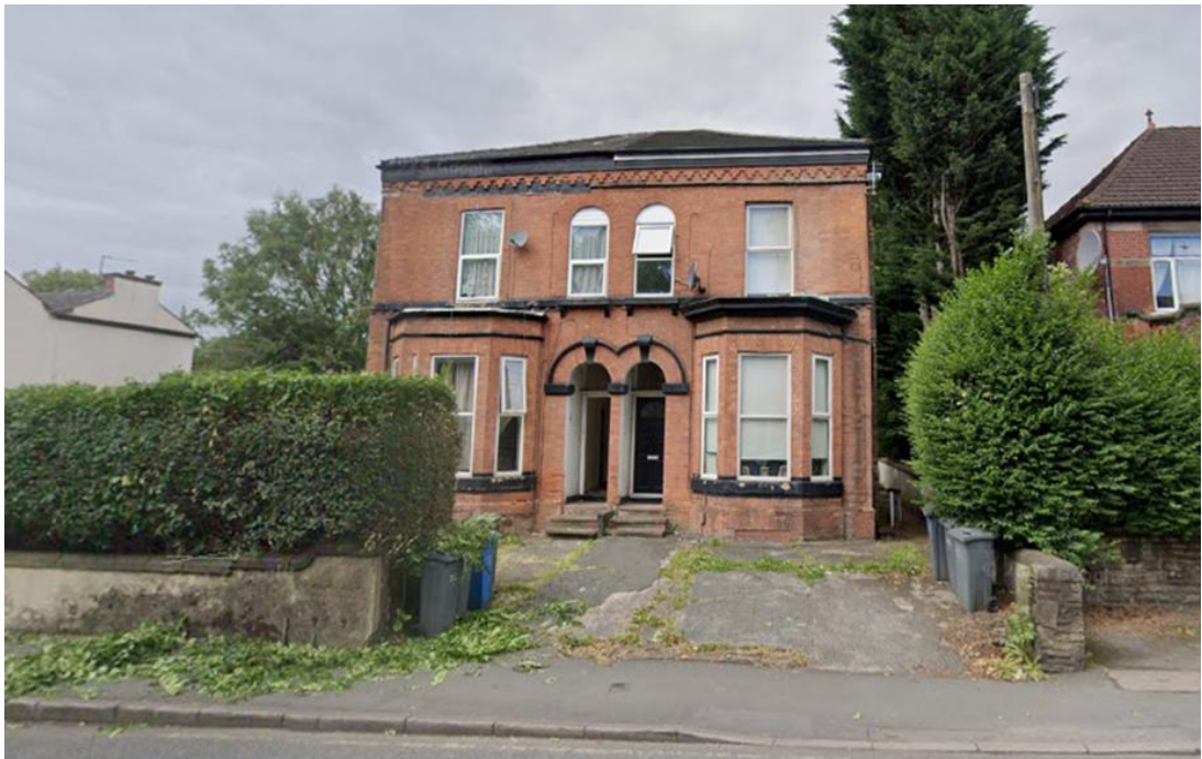
Image 1 – Streetview of front elevation of site from Middleton Street. This view demonstrates the attractive brick frontage of the Villas which respond in a positive manner to the Conservation Area.
