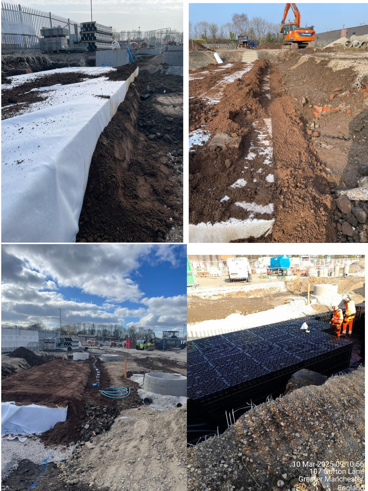
Figure 3 - Attenuation Tank Installation Phase 2 – Tank 2
