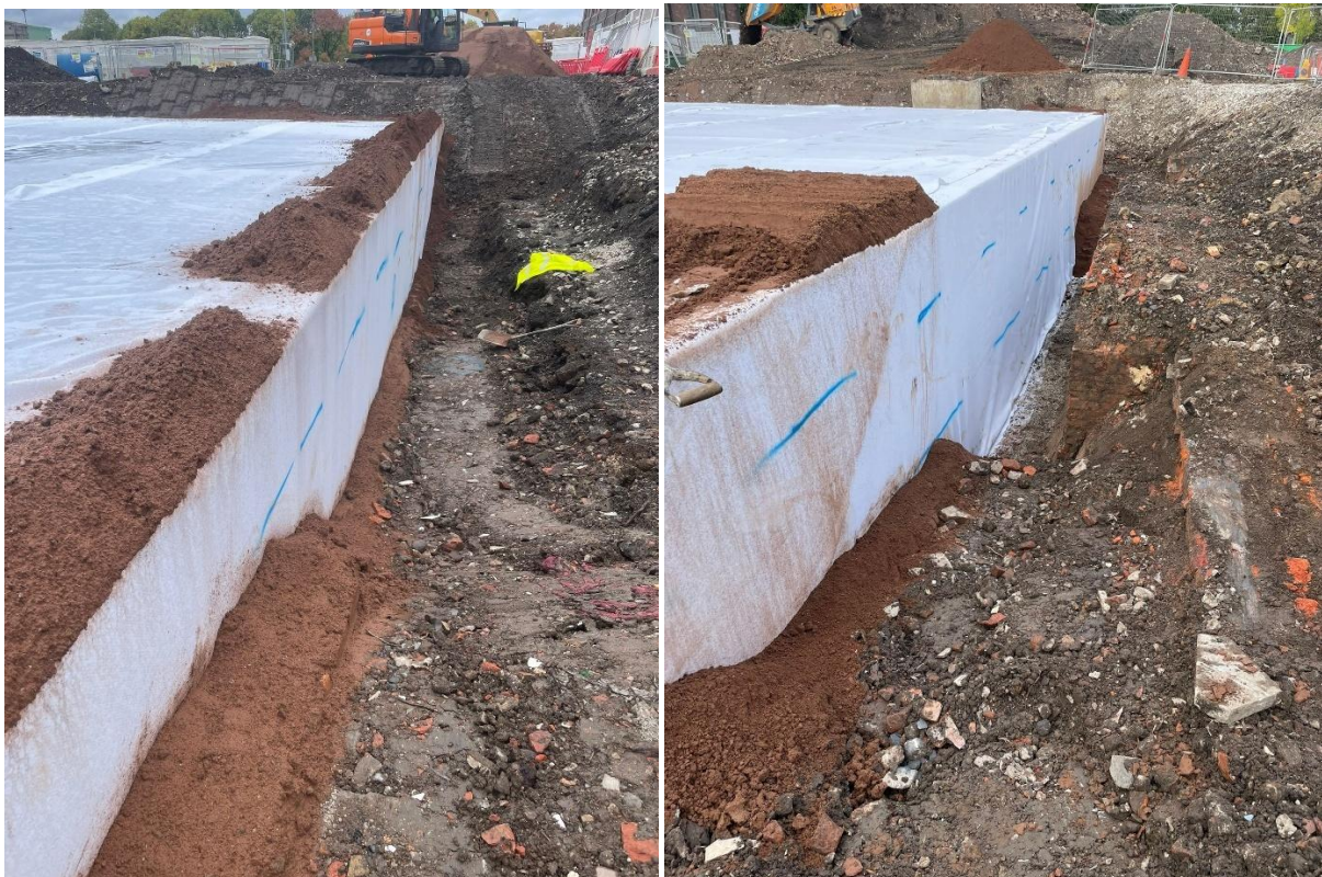
Figure 2 - Attenuation Tank Installation Phase 1 – Tank 1
