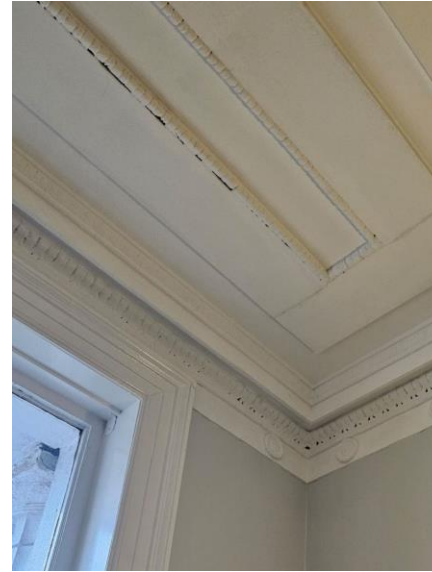
Figure 16: Coricing to Room G.007a
