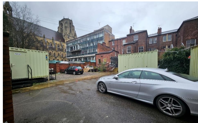
Rear of the building
