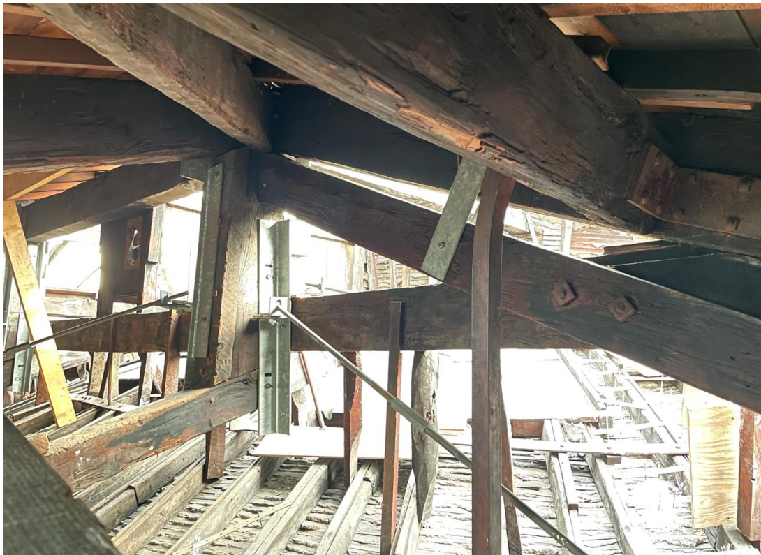
Figure 3.6 Roof truss, tension rods and dome ceiling
