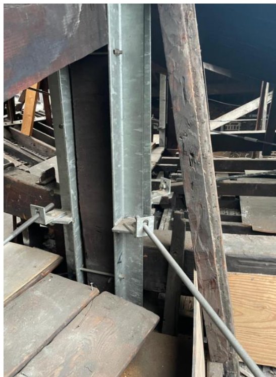
Figure 3.8 Steel rod fixing detail to the angle
