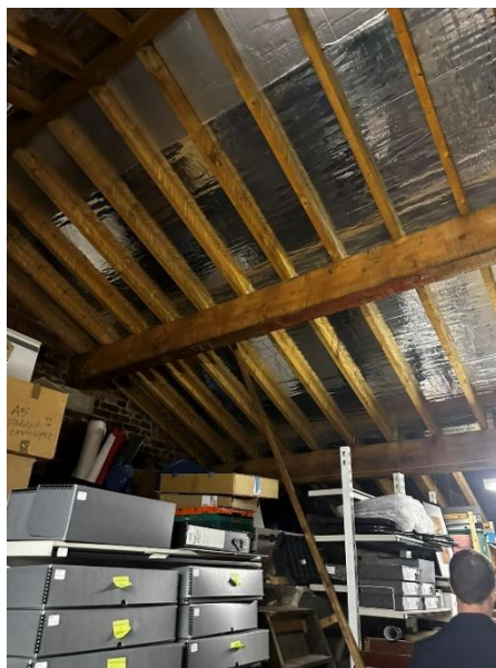
Figure 3.4 Roof space showing rafter and purlin arrangement., 2024
