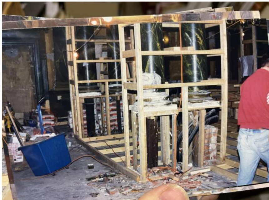
Figure 3.14 – Archive photograph showing column bases at ground floor stripped from cladding.
