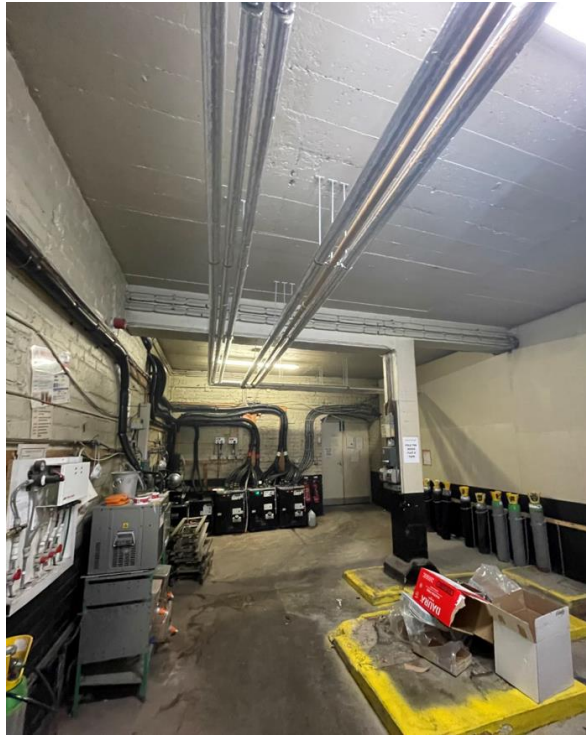
Figure 3.15 – Underside of ground floor slab viewed from basement.
