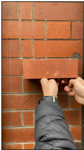
FACING BRICKS FOR WALLS (75mm Radcliffe Smooth Red by Blockley)
