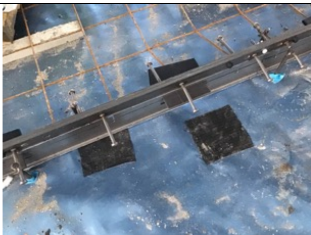
Sealed patch repairs
