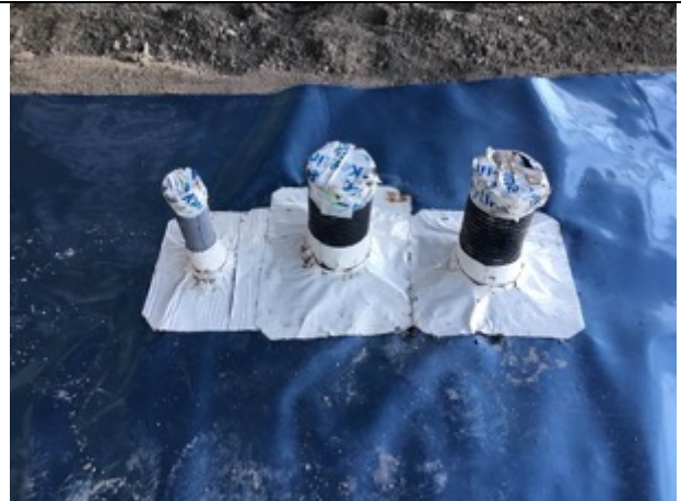
Core 6 sealed pipe penetrations
