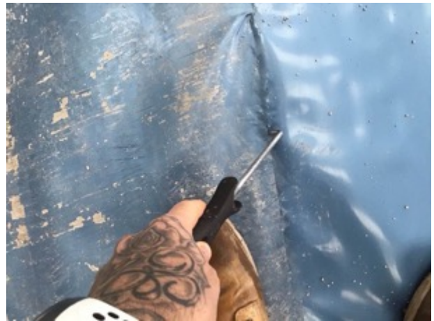
Probe test to hand welds
