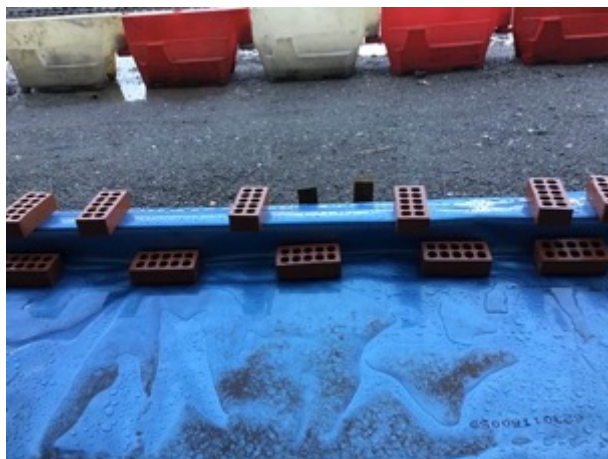
Unit 3 membrane extended over the perimeter edge
