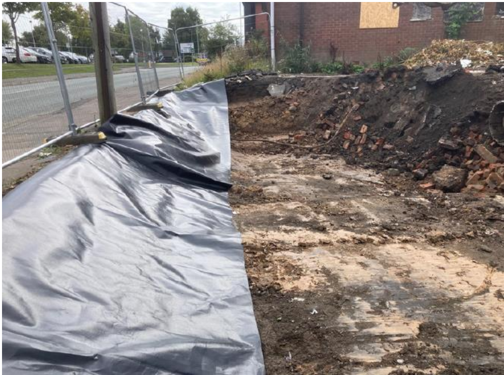
Figure 0-2 JK area 4 Excavations and barrier install to public footpath
