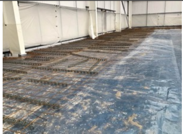
Membrane install prior to laser screed
