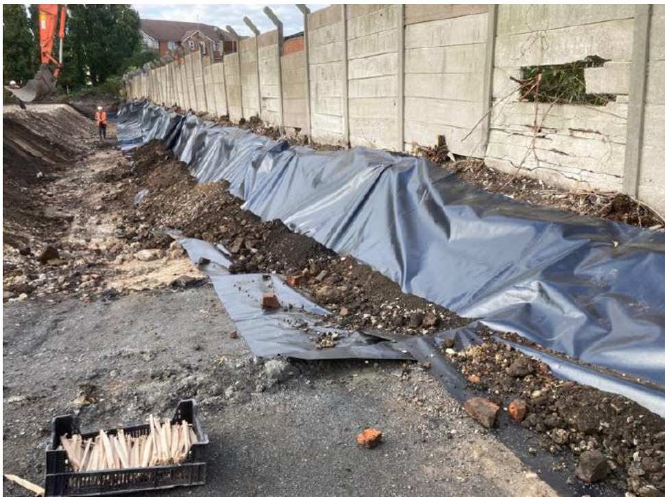
Figure 0-1 root barrier membrane installed to the northern boundary
