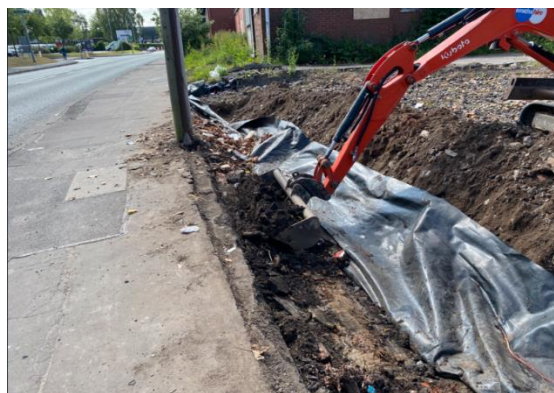
Figure 5: Removal of material from in front of the root barrier (01/06/23)
