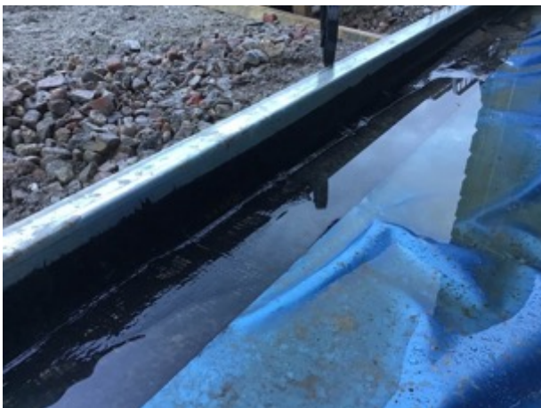
Sealed perimeter retro fit detailing
