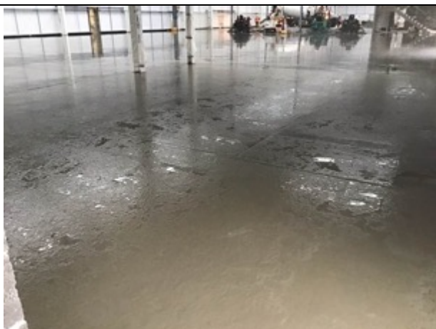
Poured under crotch area
