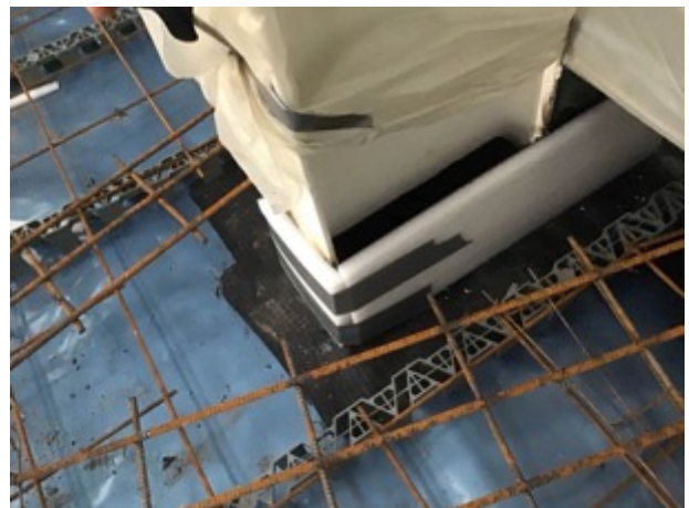
Sealed stanchion detailing
