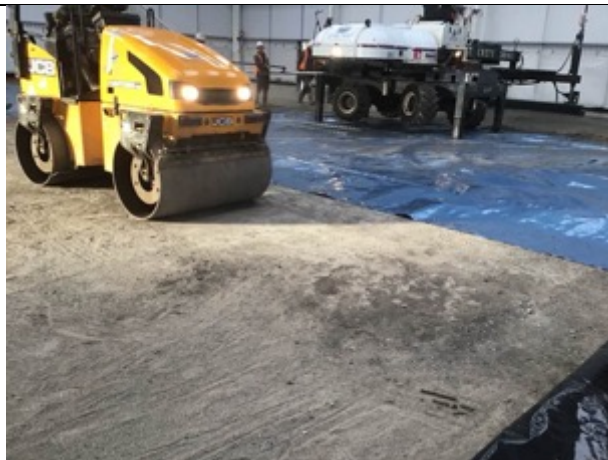
Sub grade prep
