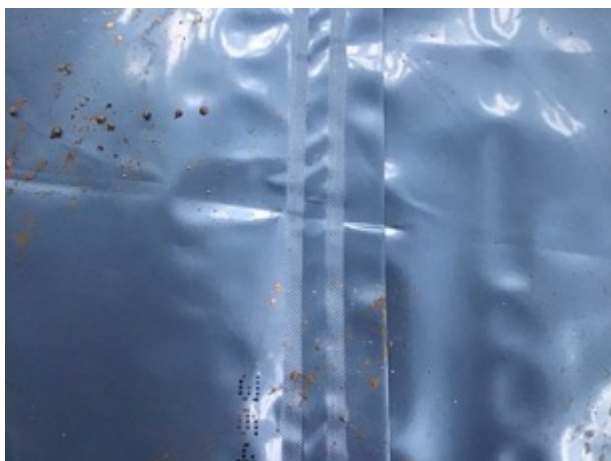
Sealed auto weld membrane joint
