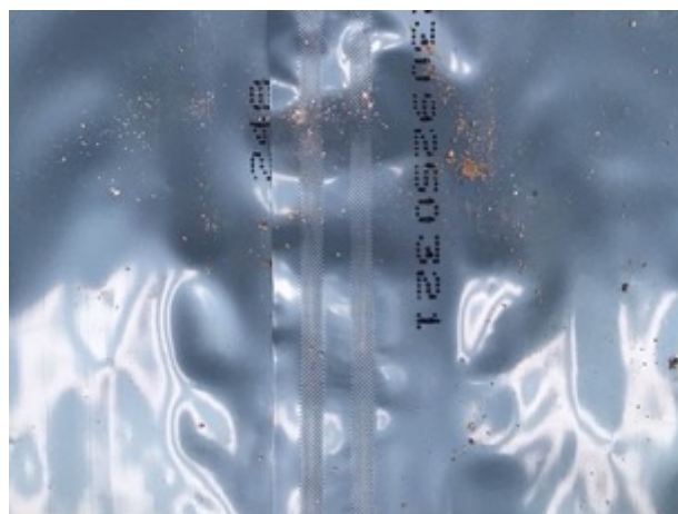
Auto weld membrane joint
