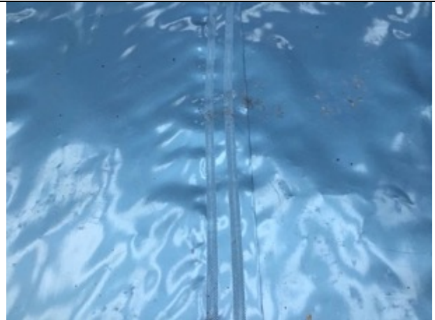
Auto weld membrane joint
