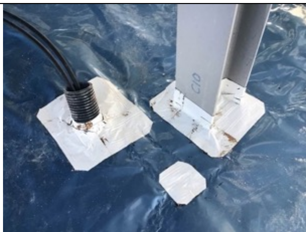
Core 8 sealed stanchion detailing, pipe penetration and patch repair
