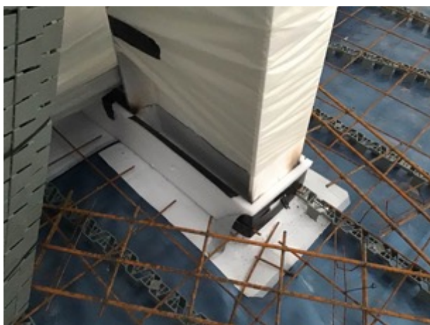
Sealed stanchion detailing
