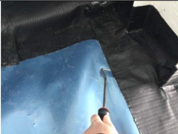
Pick testing to the SAGM detail.
