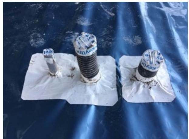
Core 5 sealed pipe penetrations
