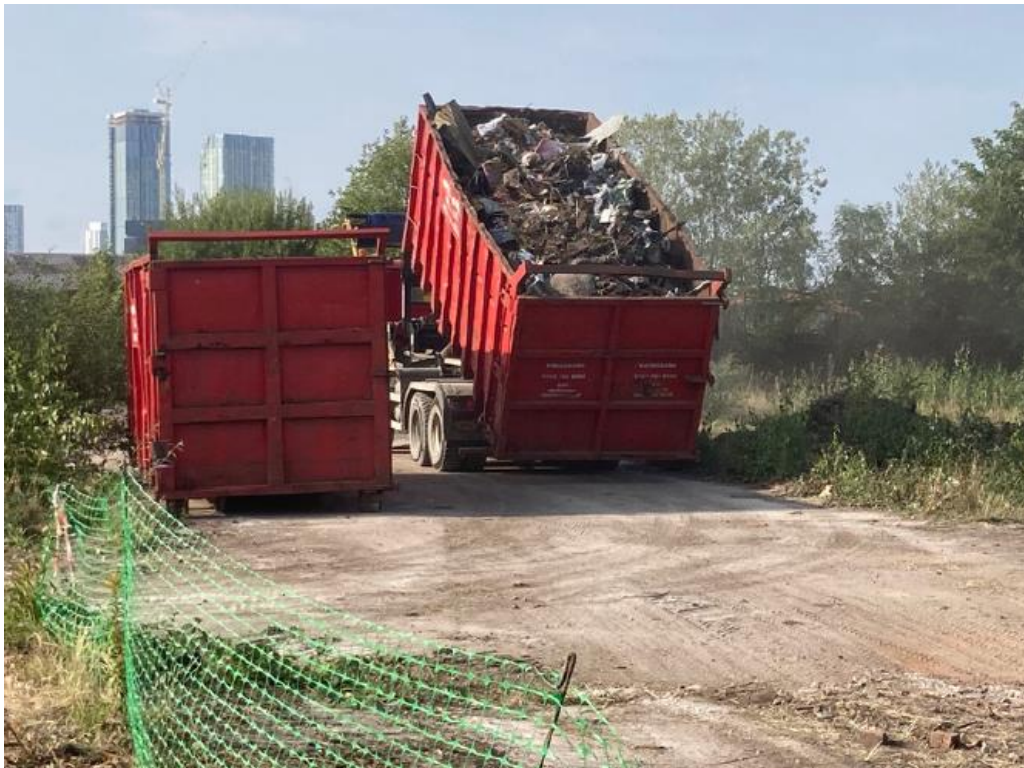
Figure 0-4 40-yard RO-RO skips removing segregated waste
