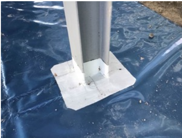
Core 6 sealed stanchion detailing
