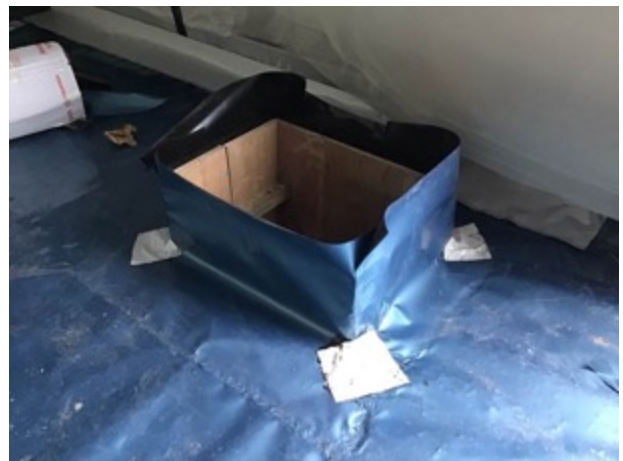
Unit 3 boxed out area
