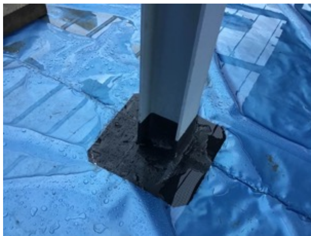
Unit 2 sealed stanchion detailing
