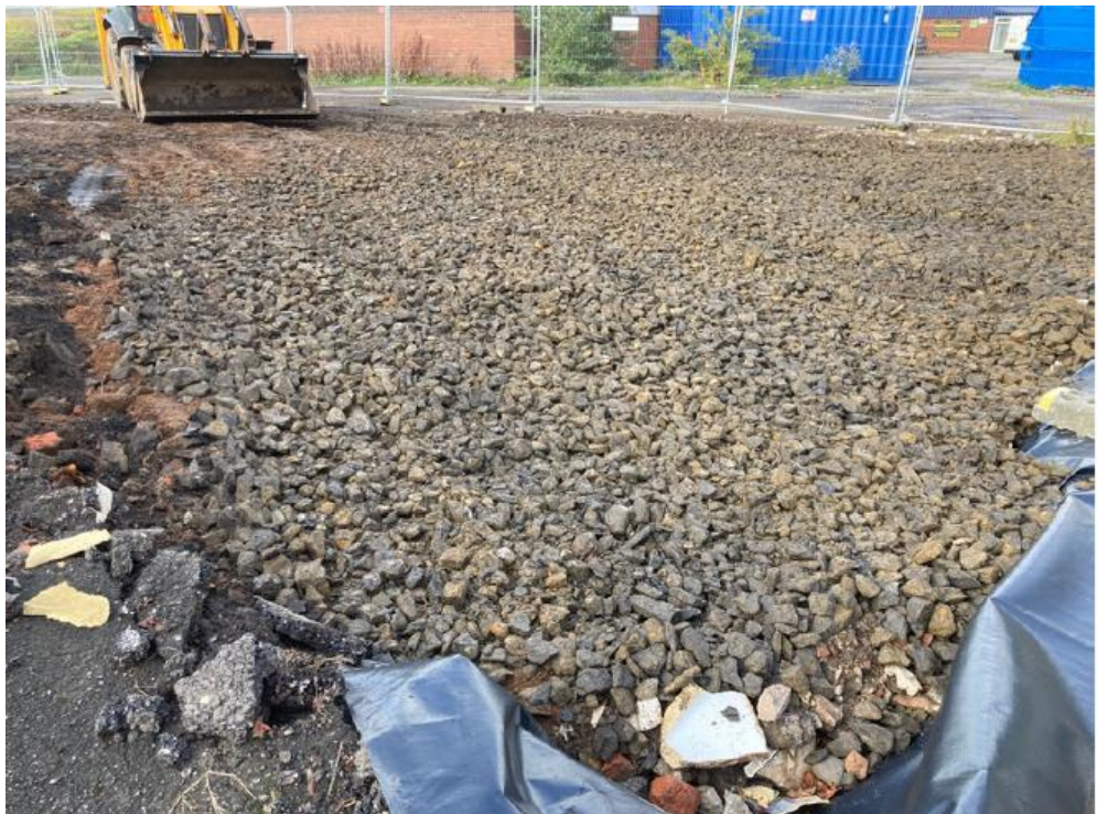
Figure 0-1 JK area 4 now backfilled with clean imported stone
