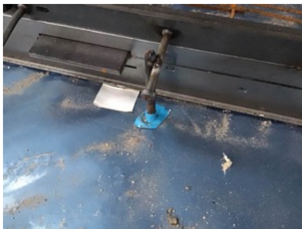
Butyl tape on armoured joint pin
