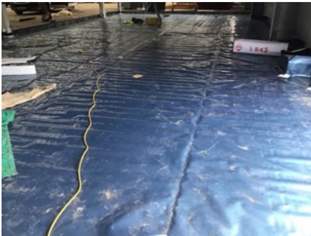
Unit 3 undercroft overview
