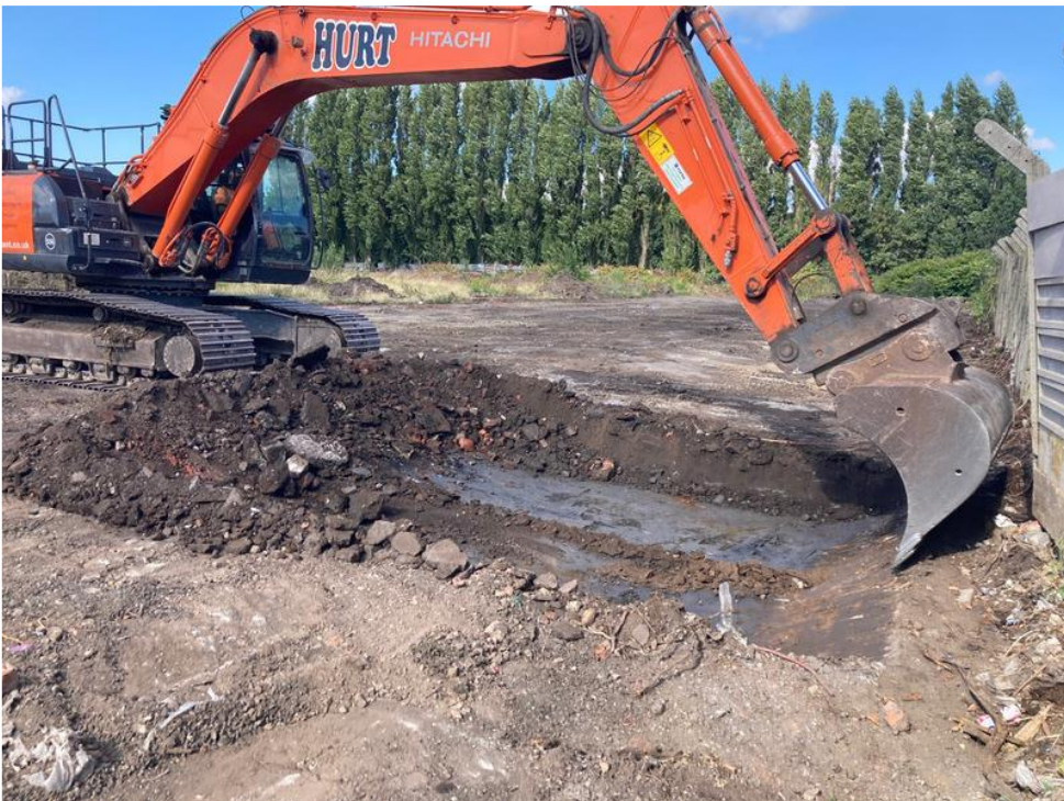
Figure 0-2Excavtions began along the northern boundary
