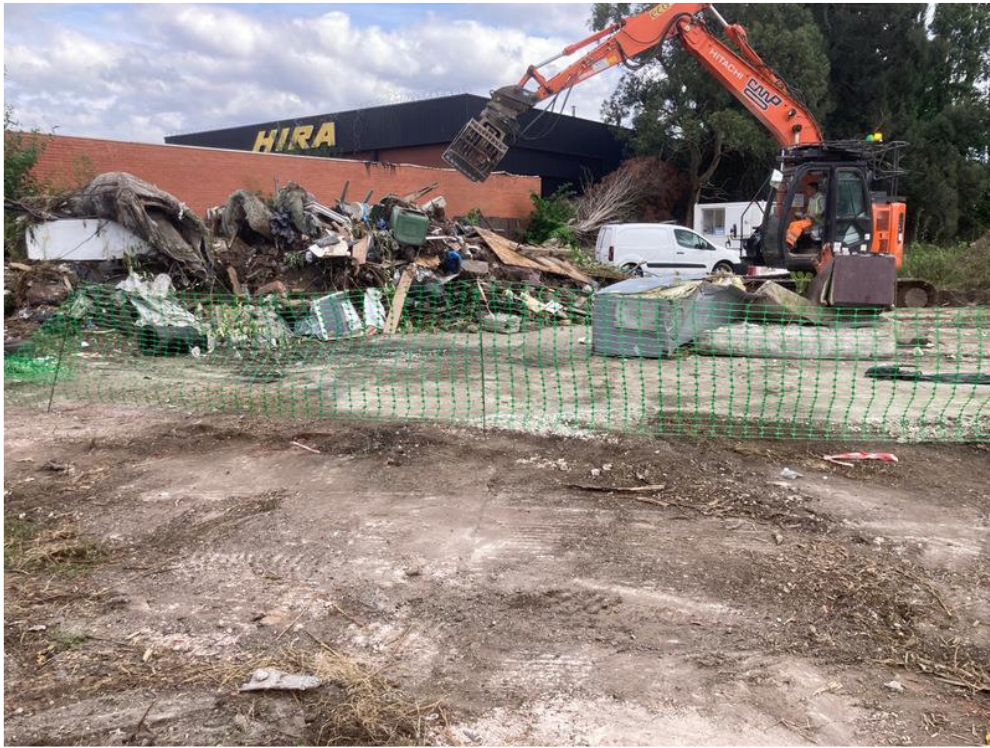
Figure 0-3 Utilising a selector grab attachment waste streams created
