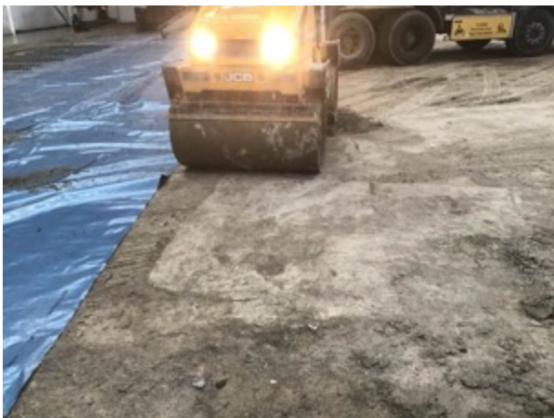
Sub grade prep
