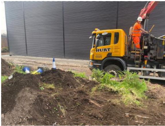
Figure 10: Excavation of Japanese knotweed (May 2024)
