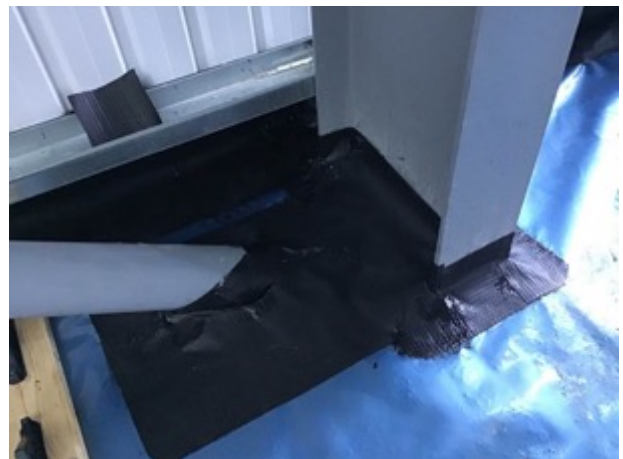
Sealed stanchion detailing
