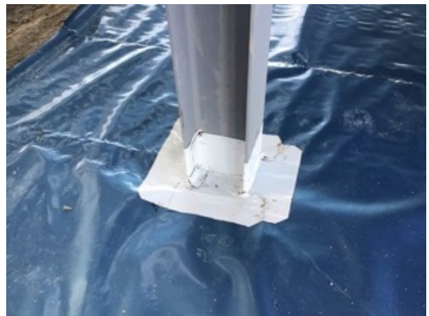
Core 7 sealed stanchion detailing
