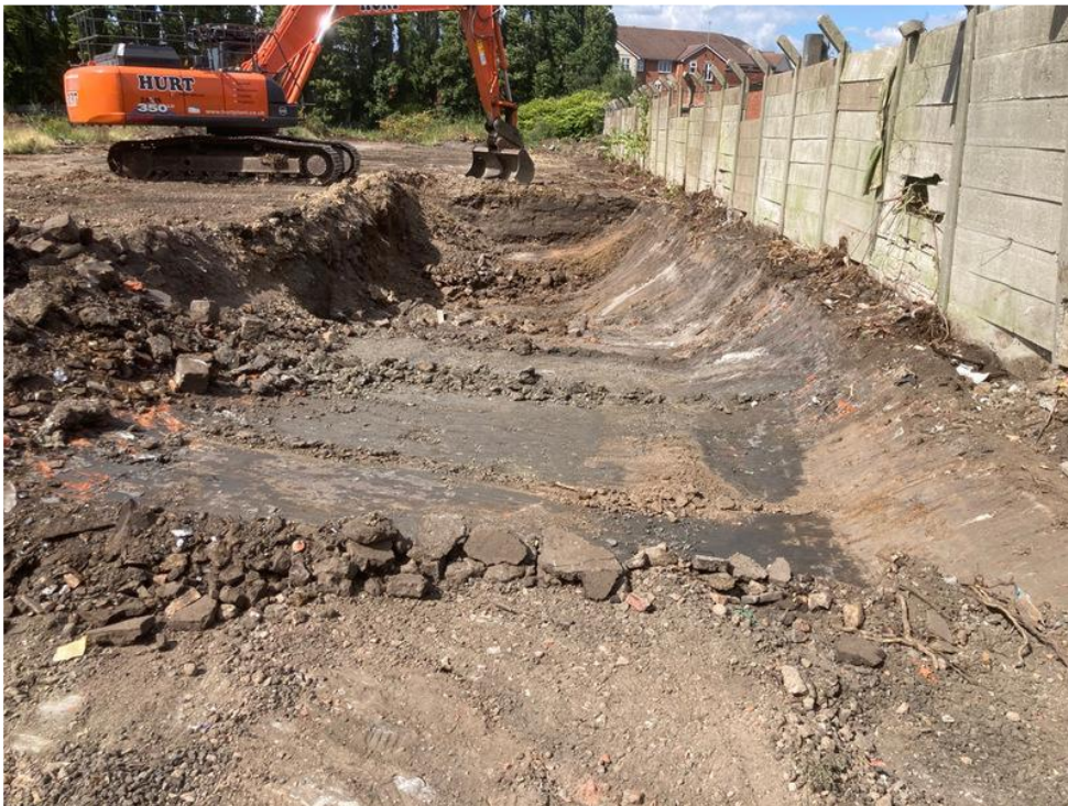
Figure 0-1 Northern boundary excavations
