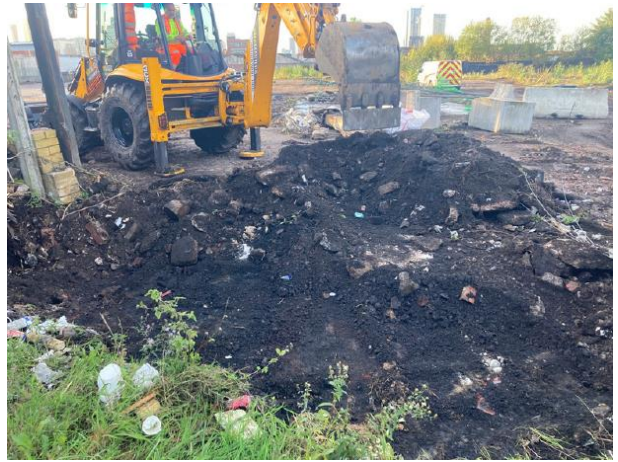
Figure 2: Excavation of regrowth (17/10/22)
