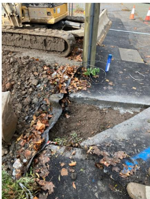
Figure 6: Uncovering the root barrier membrane (November 2023)
