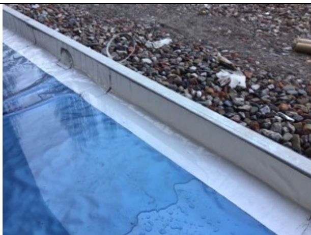
Core 8 sealed perimeter retro fit detailing
