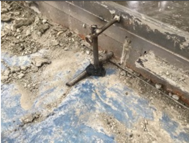
Butyl tape on armoured joint pin
