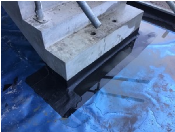
Sealed retro fit detailing to stairs
