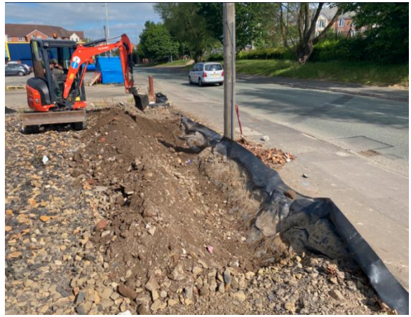
Figure 4: excavation of Japanese knotweed rhizome under root barrier (01/06/23)
