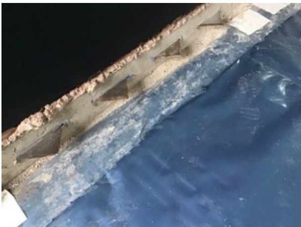
Unit 2 membrane sealed to core area existing membrane
