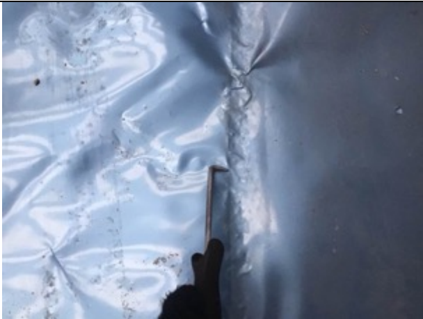
Pick test to hand weld
