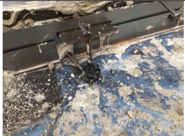
Butyl tape around armoured joint pin
