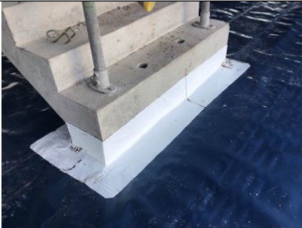
Core 5 sealed stair detailing
