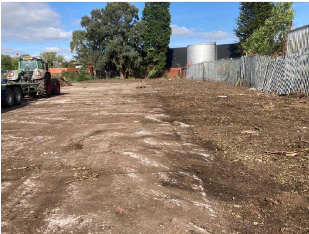
Figure 0-6 tree works and stump removal complete
