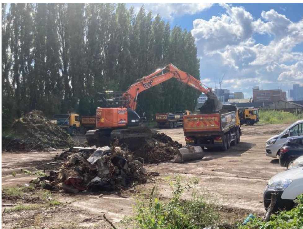
Figure 0-1 Japanese Knotweed material being loaded in to wagons for offsite disposal
