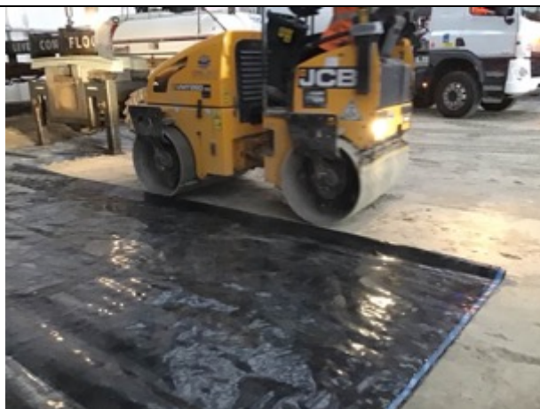
Sub grade prep ahead of the membrane installation
