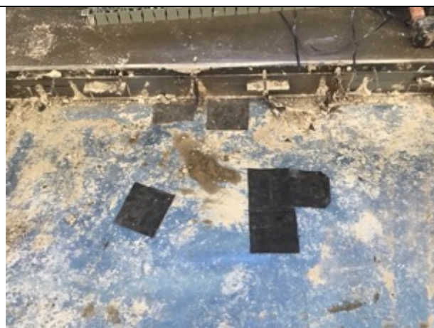
Sealed patch repairs
