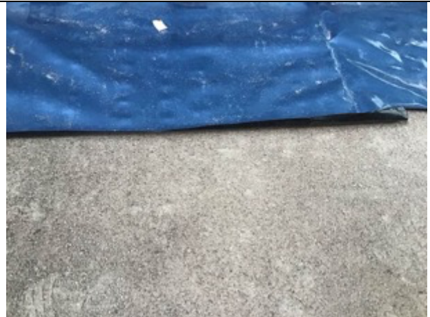
Rolled sub grade
