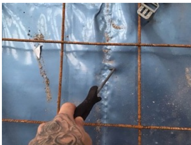
Probe test to hand weld
