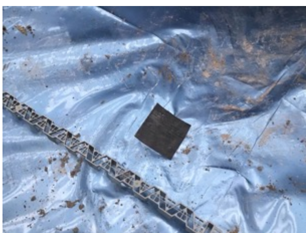
Sealed patch repair
