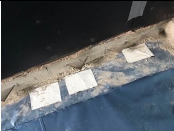
Unit 2 patch repairs
