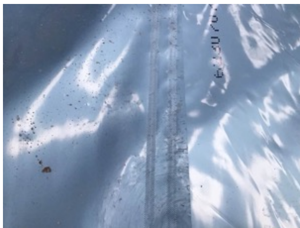
Sealed auto weld membrane joint
