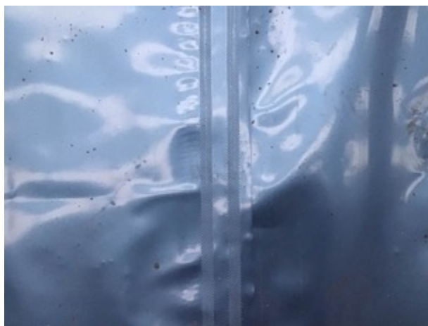
Sealed auto weld membrane joint
