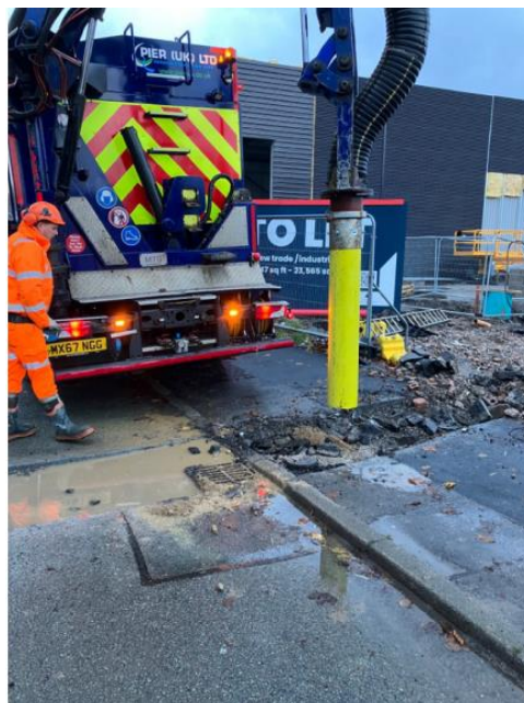
Figure 7: Vacuum excavator works (November 2023)
