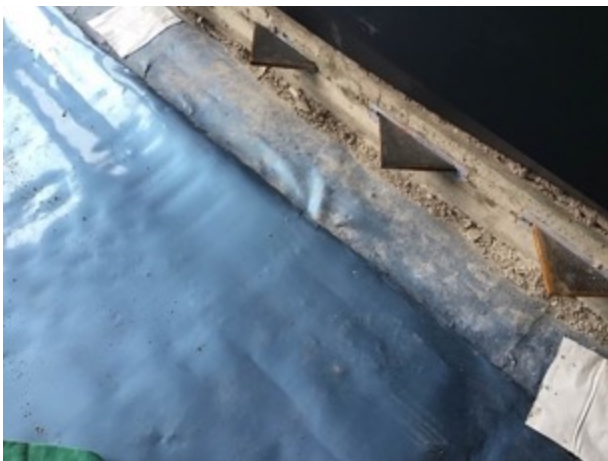
Unit 3 membrane sealed to core area existing membrane
