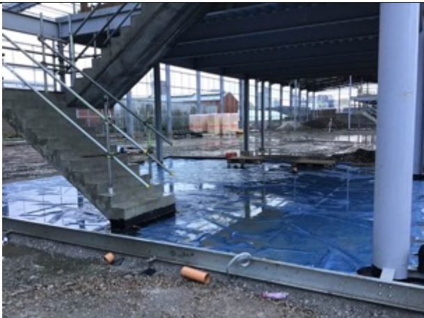
Unit 2 core area line out installation
