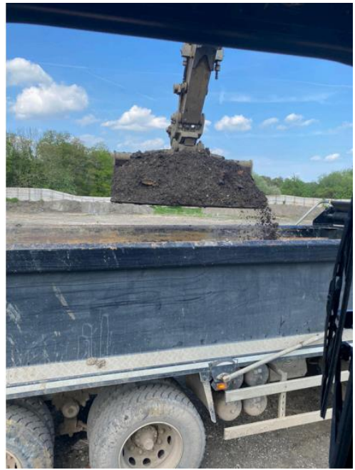
Figure 12: Loading wagons with contaminated material (May 2024)
