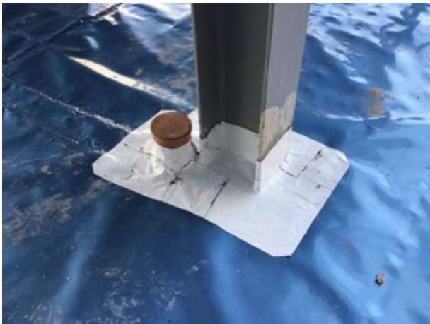
Core 4 sealed pipe penetration and stanchion detailing
