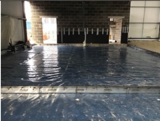
Unit 2 undercroft overview
