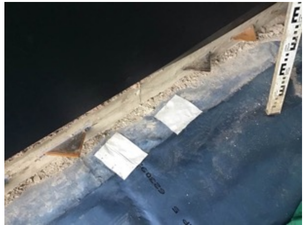
Unit 3 patch repairs
