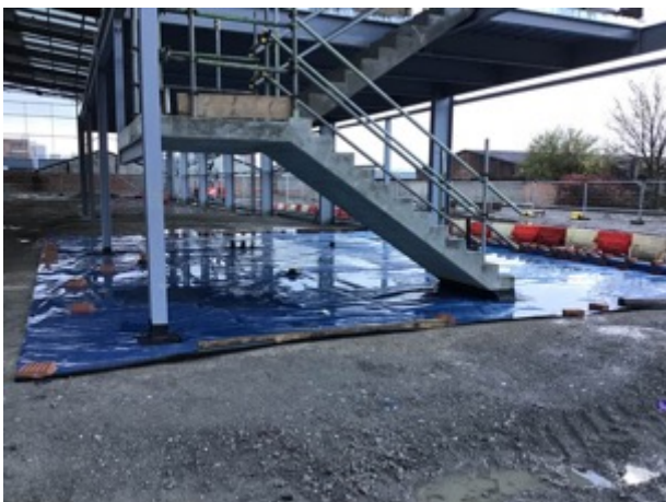
Unit 3 core area line out installation
