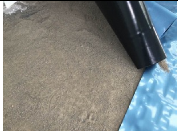
Sand blinding across the footprint within unit 1.
