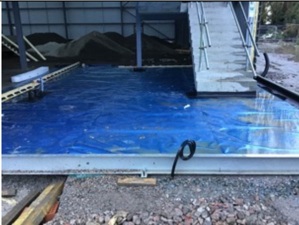
Unit 9 core area line out installation
