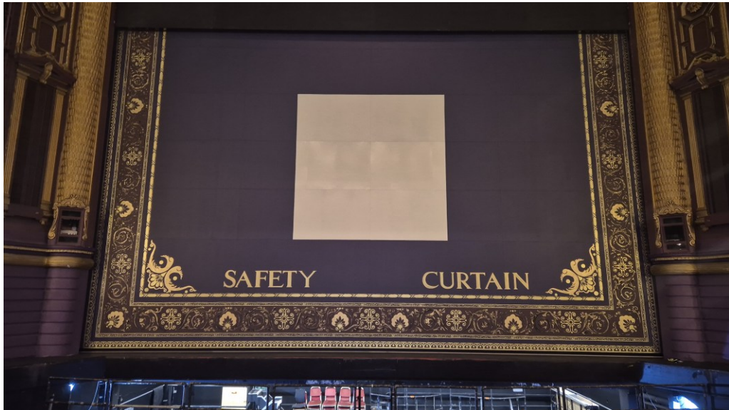
Front of new painted safety curtain.
