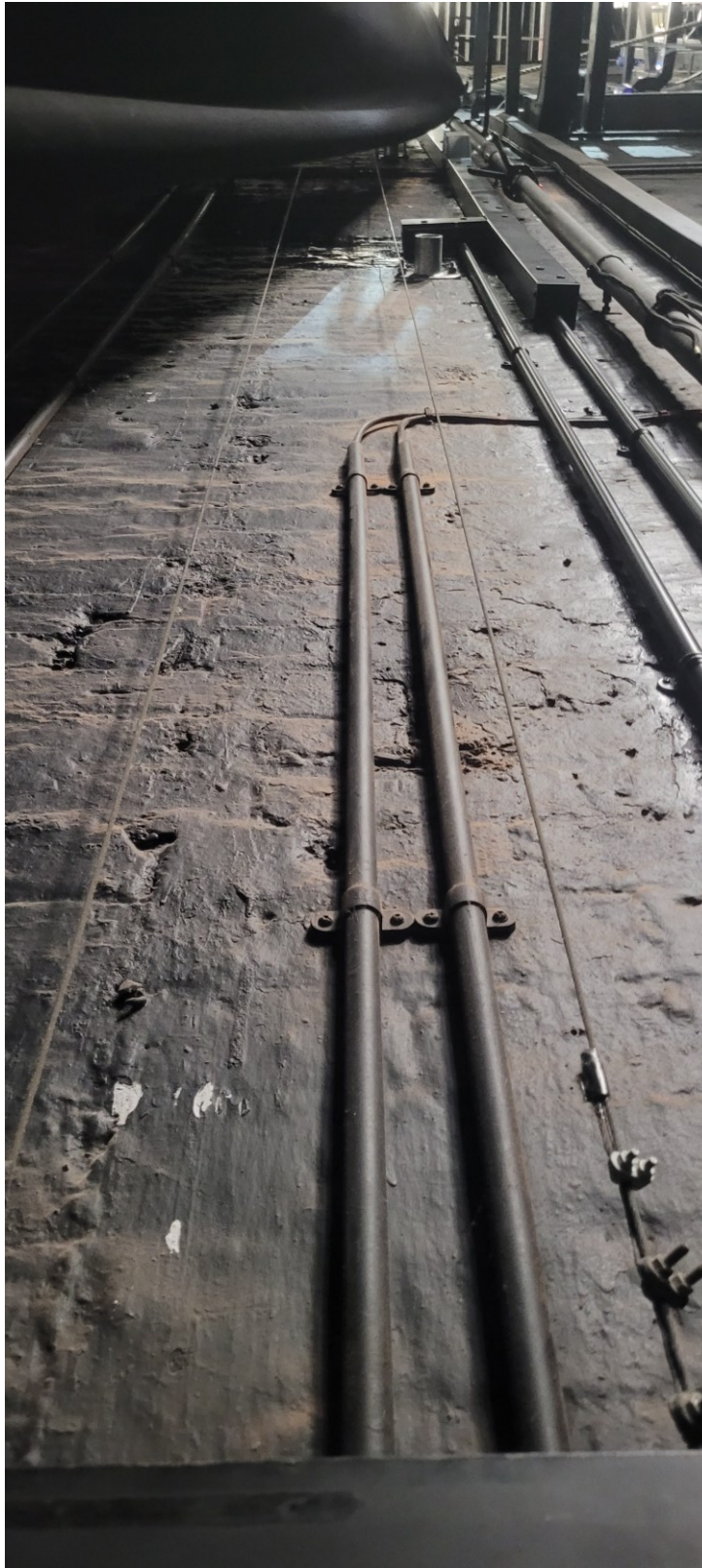
Photo 08 - Existing photograph looking up at the wall above the safety curtain control panel stage left.
