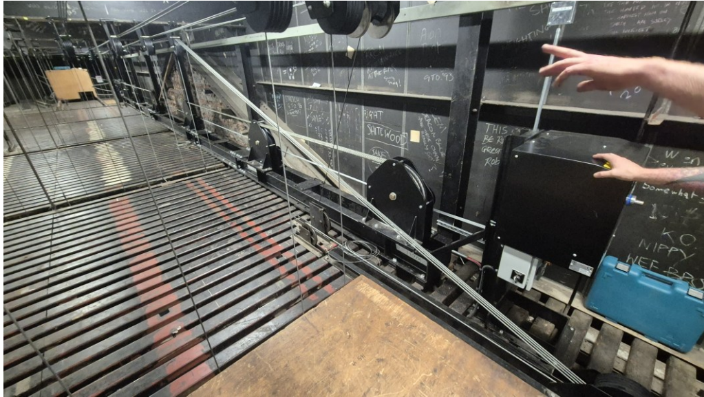
New pelmet hoist (on right) also shows new PFC's and pulleys across rear of the proscenium wall at grid level, which supports the new safety curtain and pelmet.
