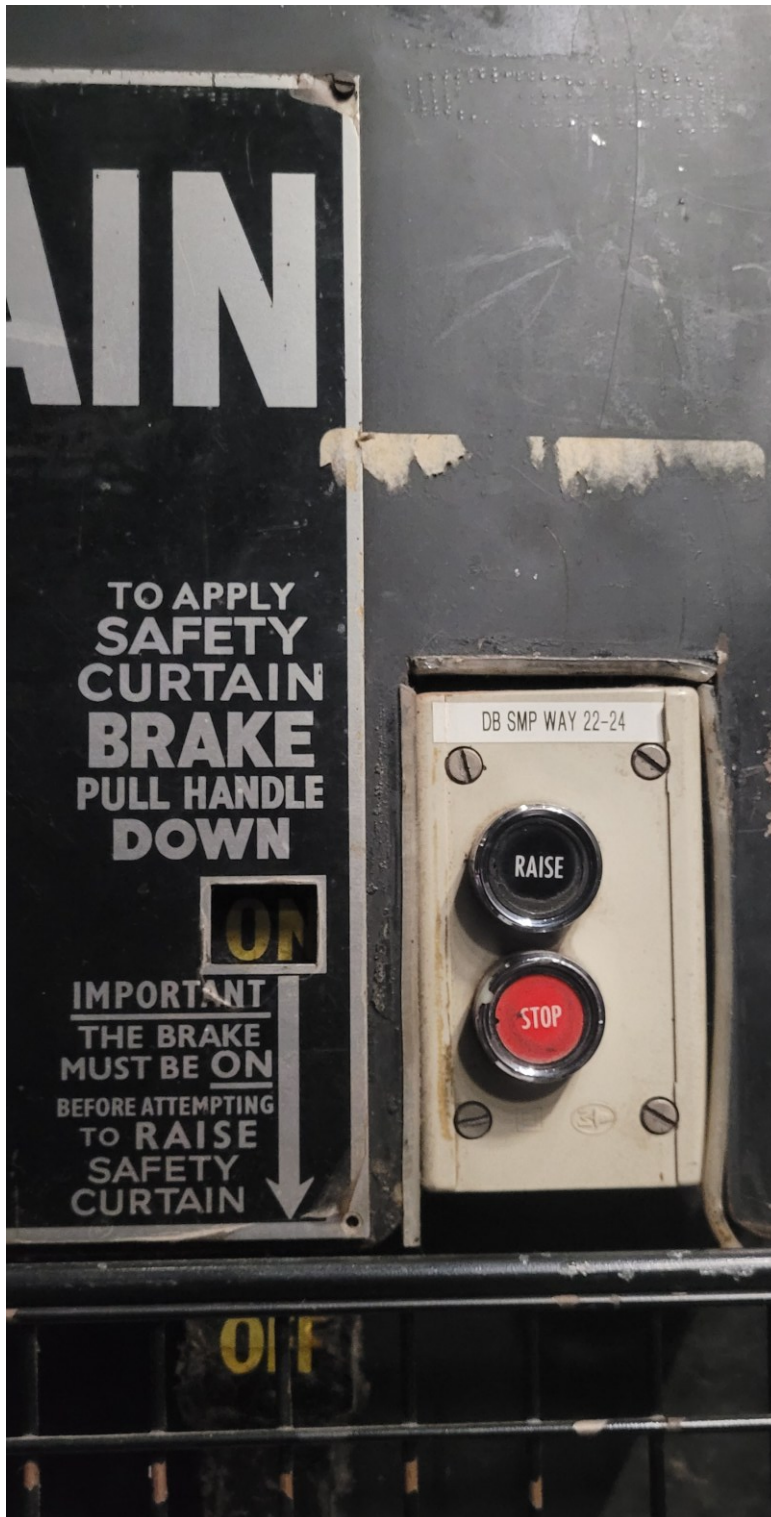
Photo 10 - Existing photograph showing close up of the safety curtain control panel stage left.
