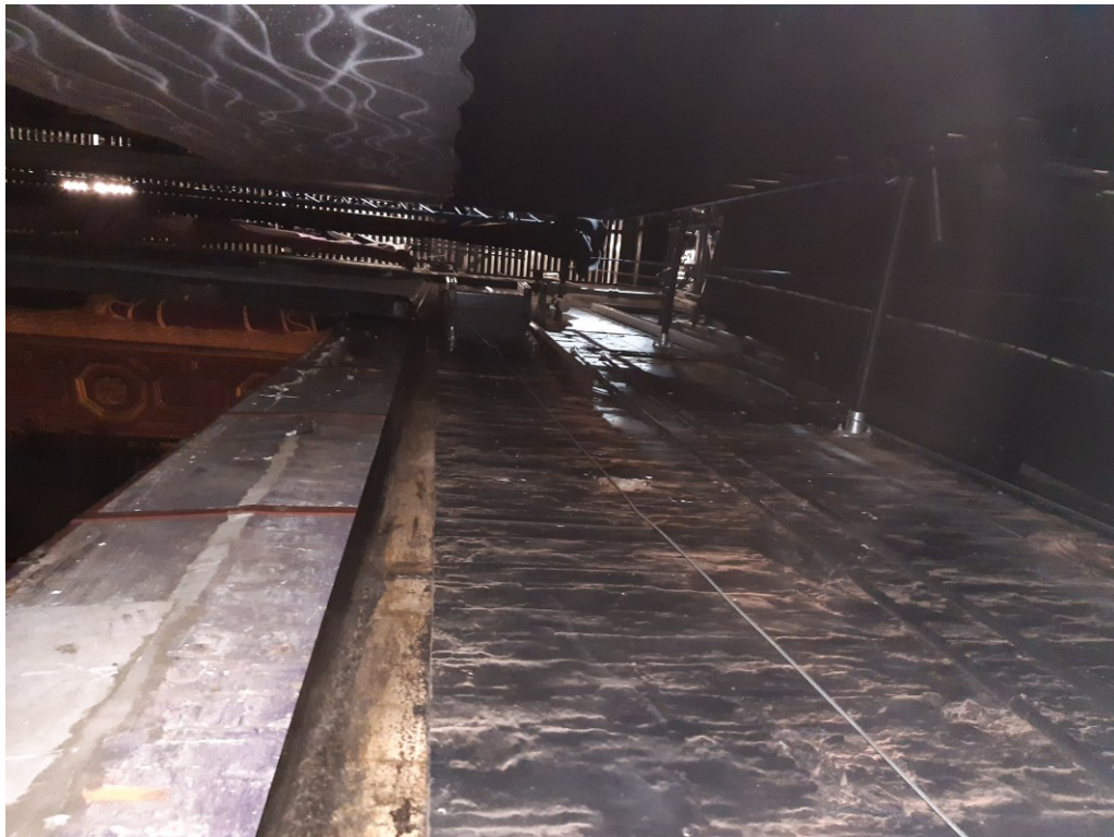
Photo 02 - Existing photograph looking up the B.O.H. wall stage left.
