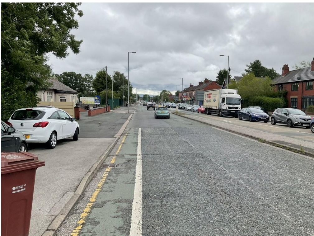
6.2 General view looking southeast on Hollinwood Avenue towards the proposed junction.
