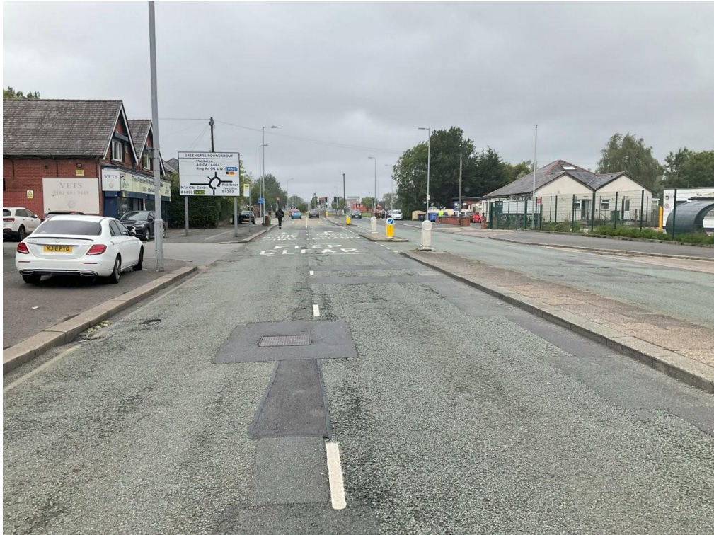
6.1 General view looking northwest on Hollinwood Avenue towards the proposed junction.
