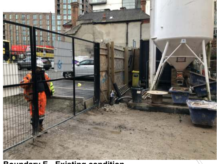
Boundary E - Existing condition Used as main access into construction site.
