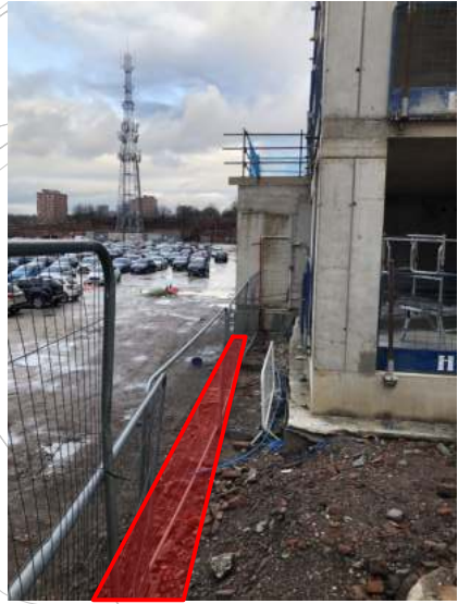
Wall A - Existing condition Demolished required rebuilding.
