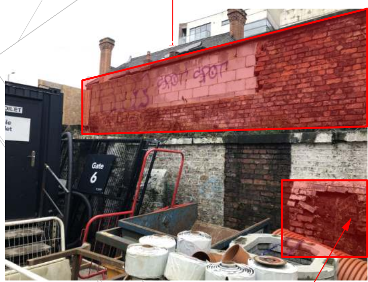
Wall D - Existing condition
