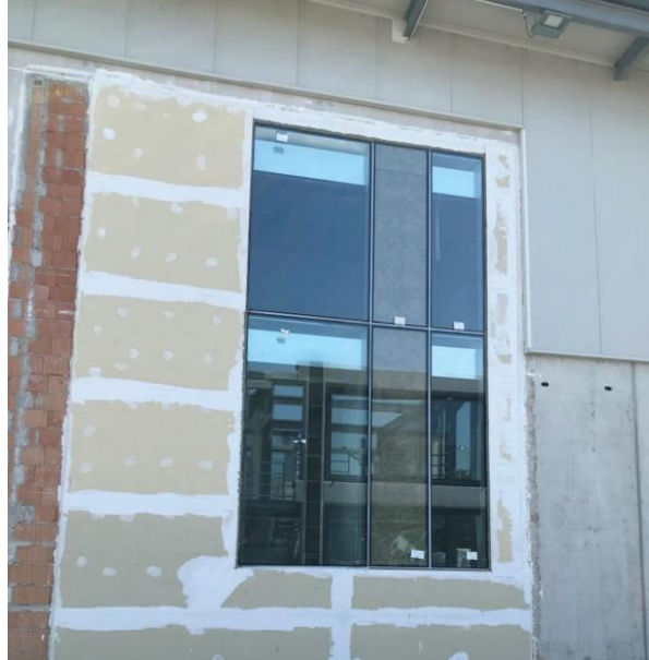
Photo 2.1 – Mock up of External Cladding
